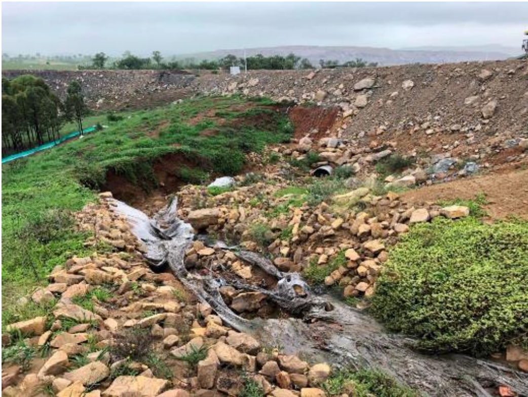
Erosion Photo 3 - Rock lined drain near the pit top has failed and needs full redesign and rework
