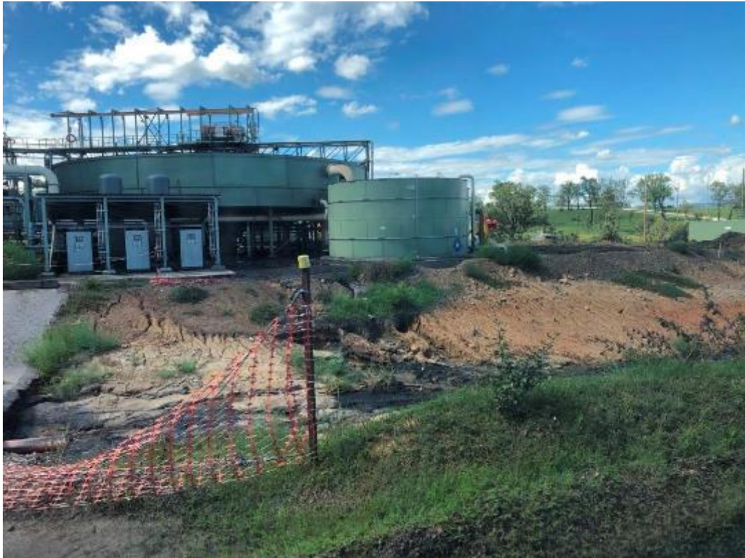
Erosion Photo 7 - Erosion in the CHPP Area. Some works have completed since the site inspection (April 2020) but ongoing maintenance is required.
