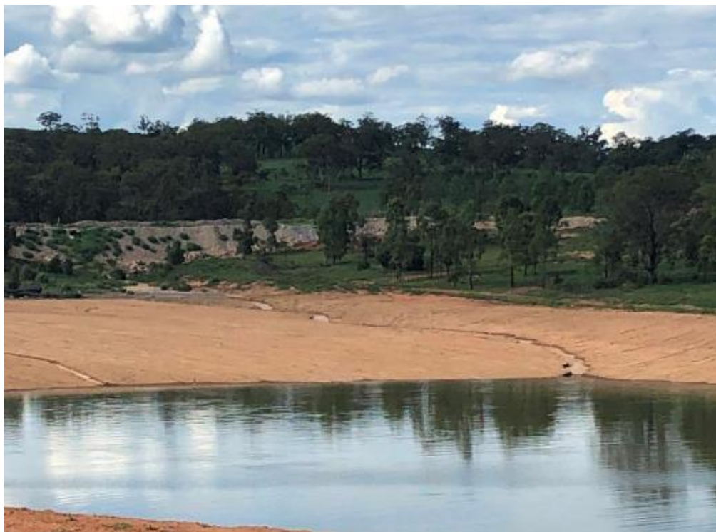
Erosion Photo 16 - Erosion in the Mine Water Dam. Since the site inspection the area has been remediated
