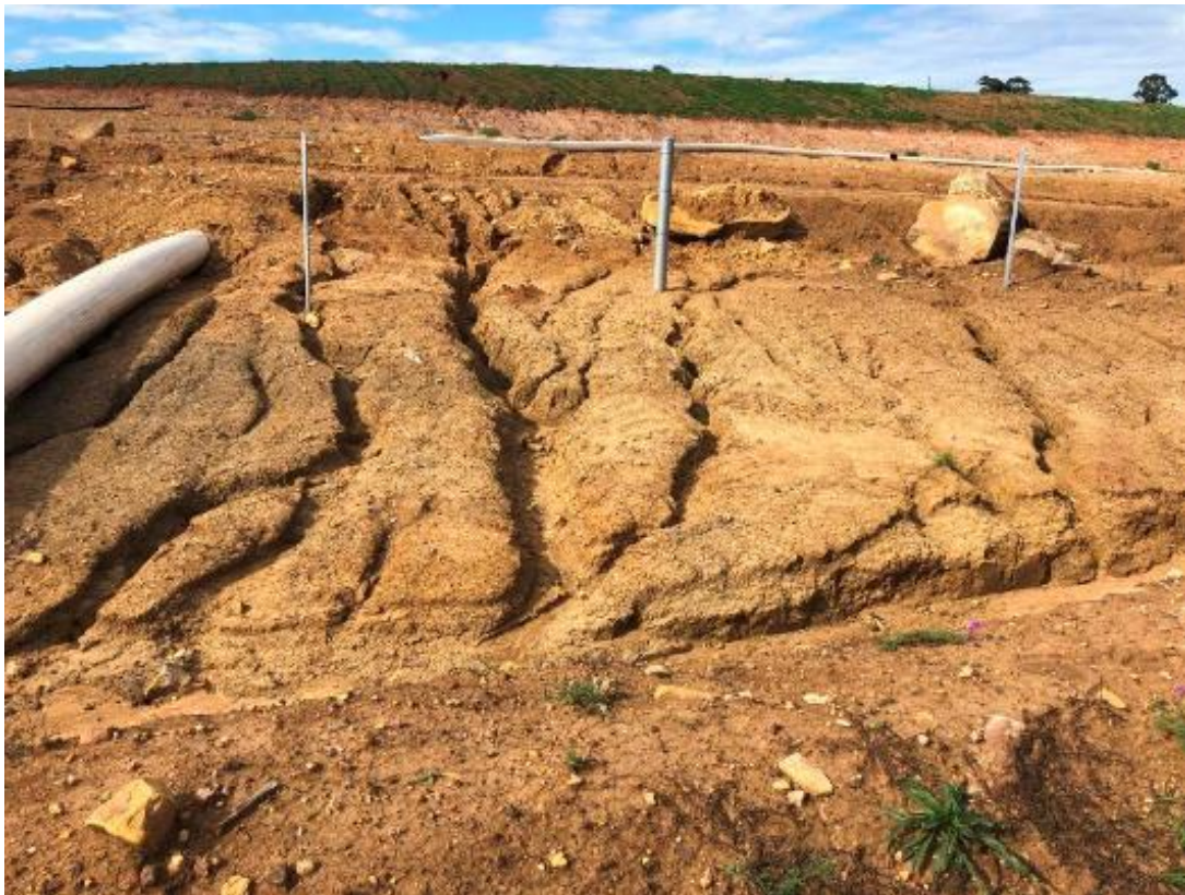
Erosion Photo 10 - Erosion within the fines emplacement area. Within the dirty water catchment.
