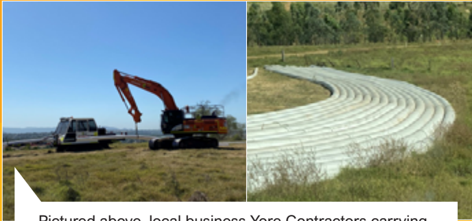
Pictured above, local business Yore Contractors carrying out pipe joining on the Rail Loop Project with the picture on the right showing the completed welded pipe.
