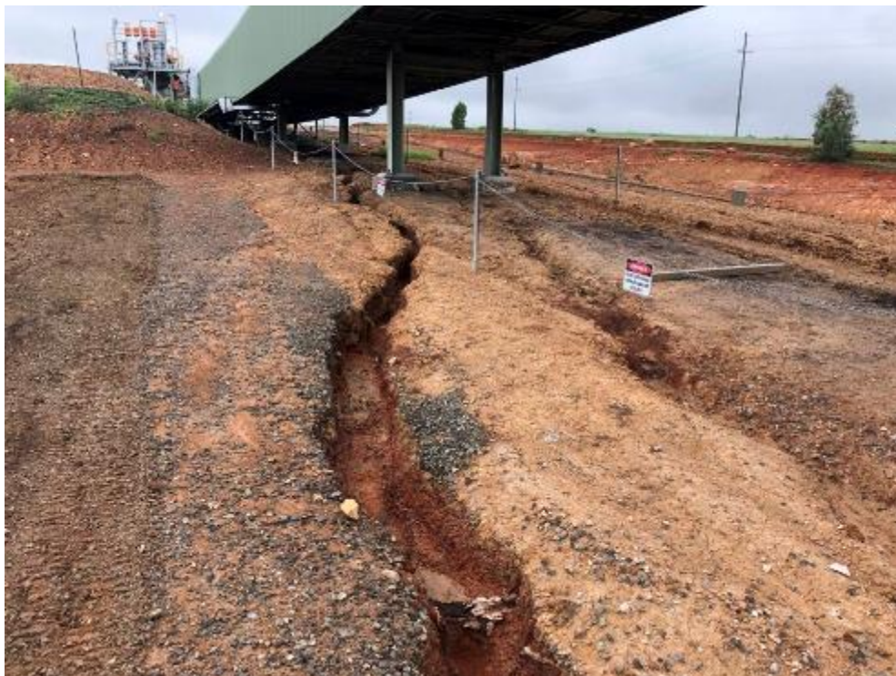
Erosion Photo 4 - Erosion along the roadway to the Train Load Out Area. Note – Evidence provided that erosion issue has been remediated, however maintenance is ongoing
