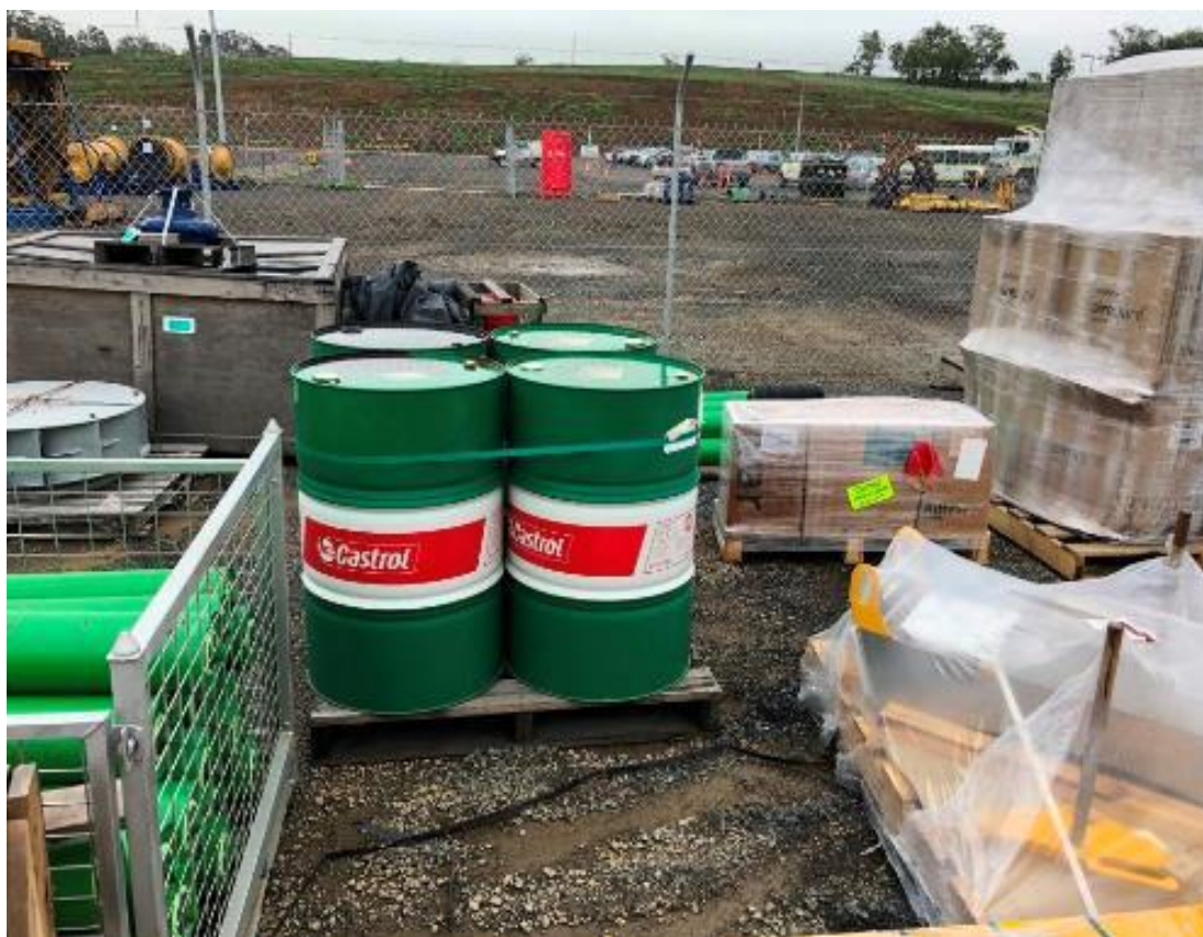
Waste Photo 6- Workshop Area. 44 gallon drums containing oil have not been stored within bunds
