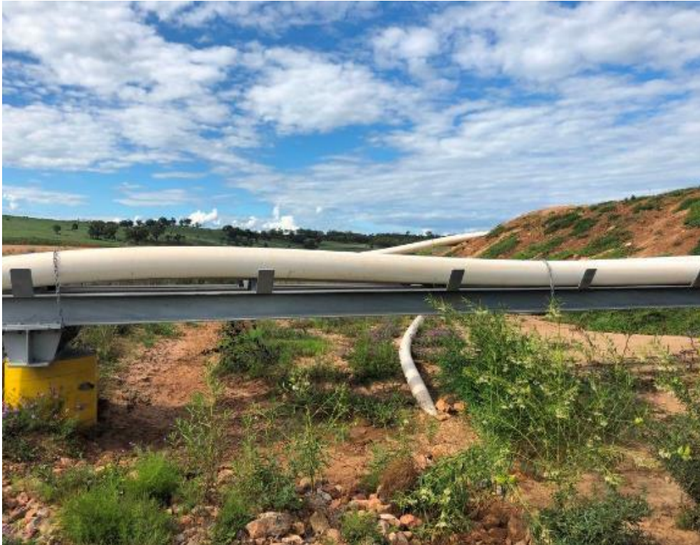
Water Management Photo 17- Fines disposal pipeline cross the cleanwater drain. Note, evidence provided since audit inspection of the installation end of line burst protection flow meters.
