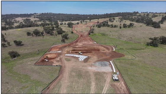
Plate 9 – Construction of Northern Link Road (September 2025)
