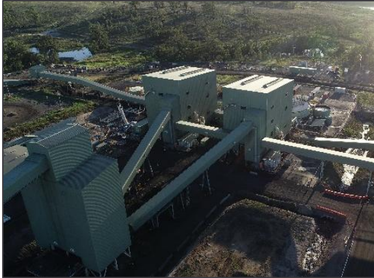
Plate 1 – Existing CHPP Modules and Materials Handling Systems
