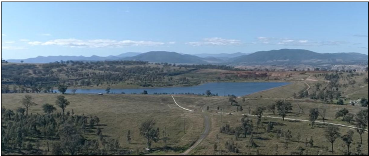
Plate 34 – Mine Water Storage Mount Pleasant Operation
