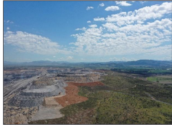
Plate 2 – View of South Pit and Eastern Out-of-Pit Emplacement (Looking North)
