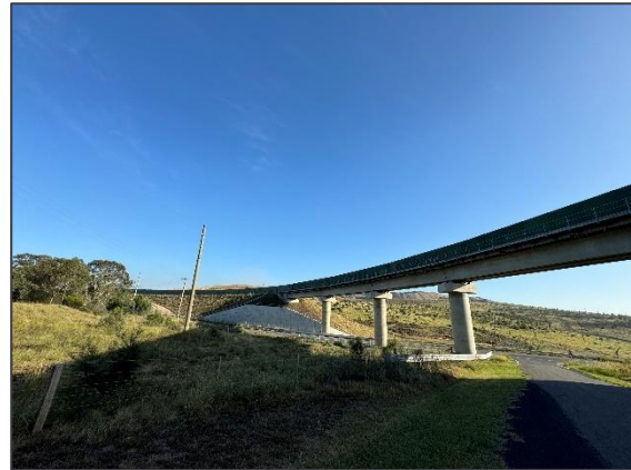
Plate 14 – Existing Stage 2 Rail Overpass of Wybong and Overton Roads
