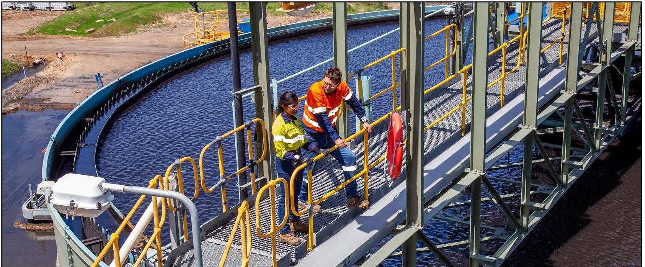
Plate 6 – Mount Pleasant Operation Coal Processing Infrastructure
