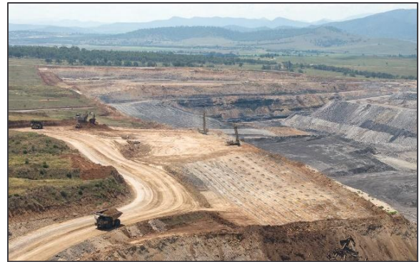
Plate 12 – Noise Attenuated Excavator and Haul Trucks Operating, Mount Pleasant Operation
