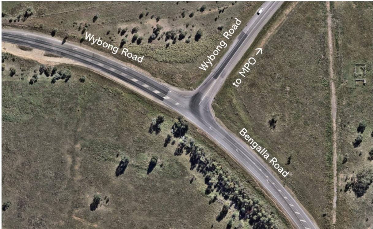
Figure 3.3: Intersection of Wybong Road and Bengalla Road
