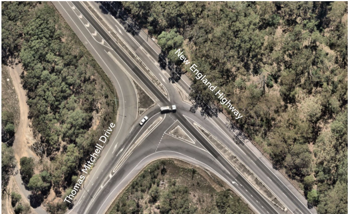
Figure 3.7: Intersection of New England Highway and Thomas Mitchell Drive
