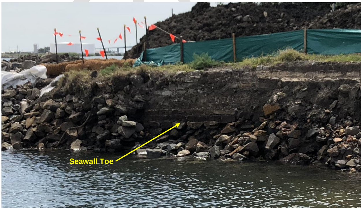
Figure 2: View of uncovered toe of heritage seawall in NE corner of Boat Harbour
