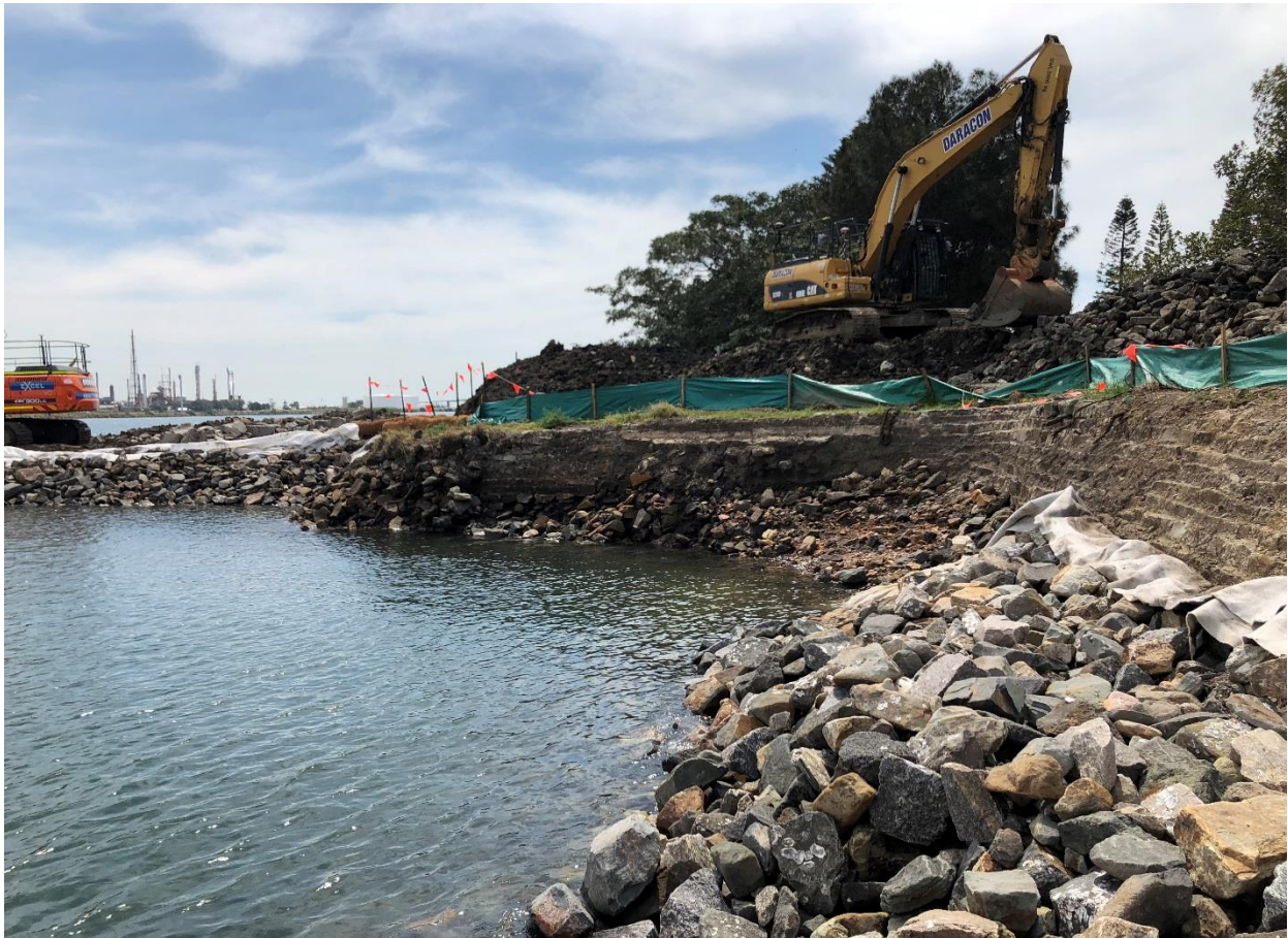
Figure 1: View looking towards NE corner showing partially built rock revetment and face of heritage seawall
