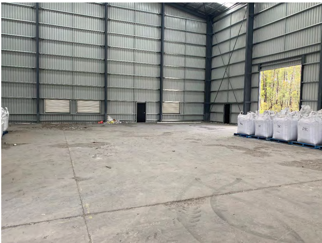
Plate 22 - Decommissioned briquetting plant
