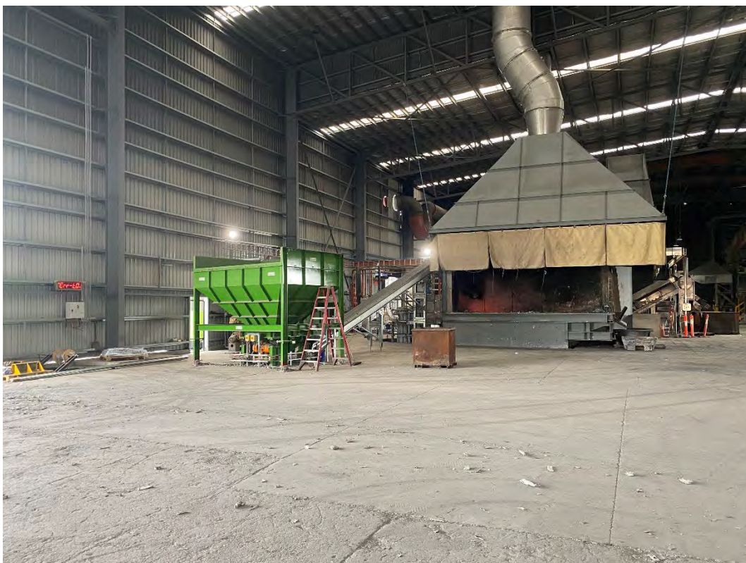
Plate 2 - Clean, dust free Plant floor
