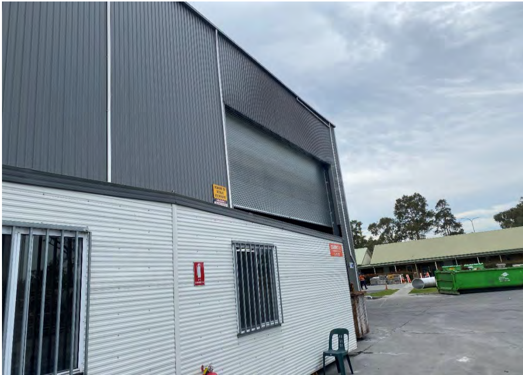
Plate 9 – Site office with partially enclosed shed door employing dust mitigation water spray
