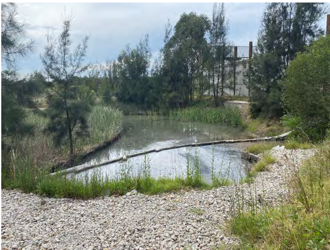
Plate 18 - Onsite stormwater containment dam
