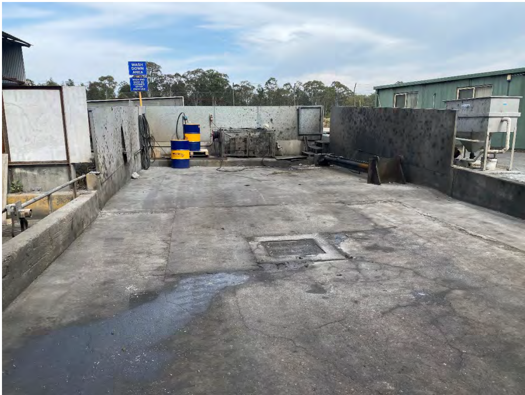
Plate 15 - Wash down area with oil separator in background
