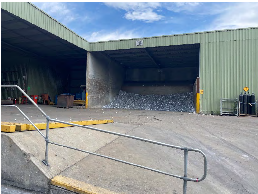
Plate 8 – Puck storage area
