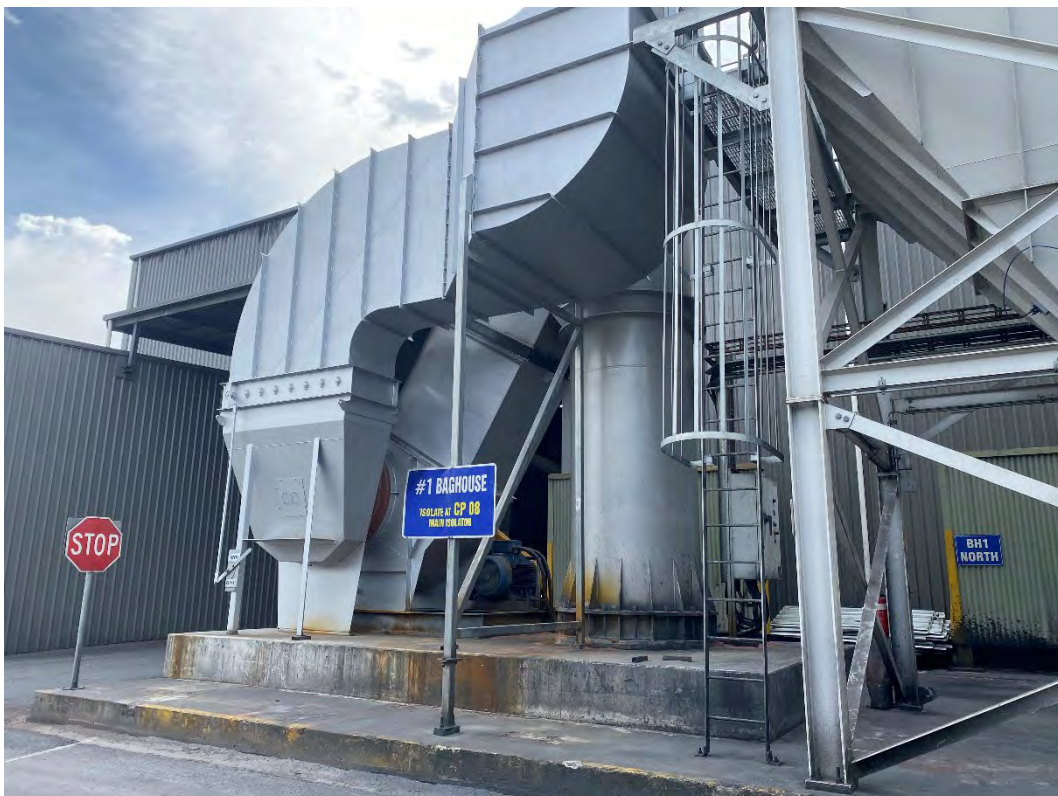
Plate 12 – Baghouse No. 1 with traffic control signage in foreground
