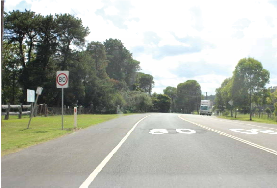
Photograph 6.6 Menangle Road 1.5 km north of Station Street looking north
