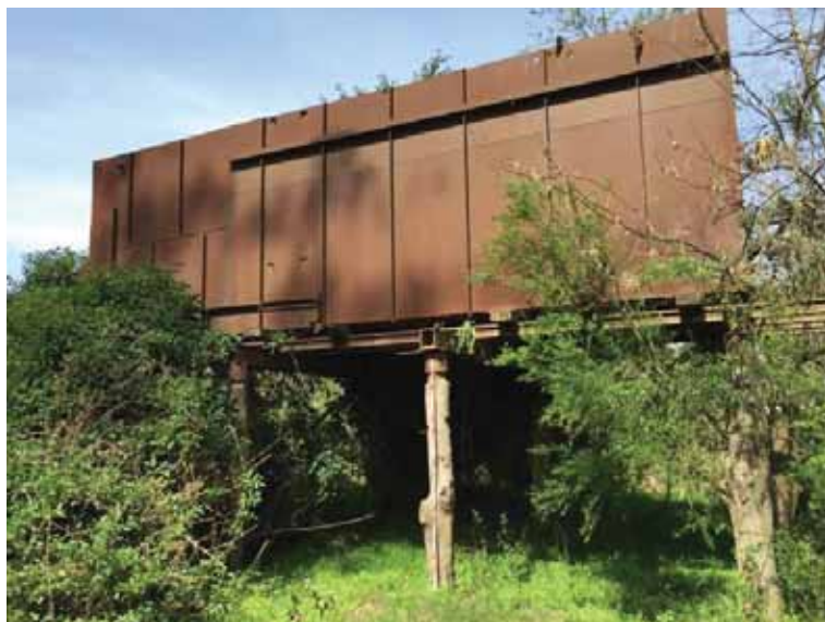
Photograph 6.1 Storage container west elevation
