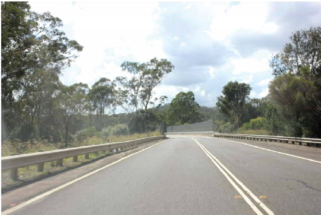
Photograph 6.7 Menangle Road 3.5 km north of Station Street looking north
