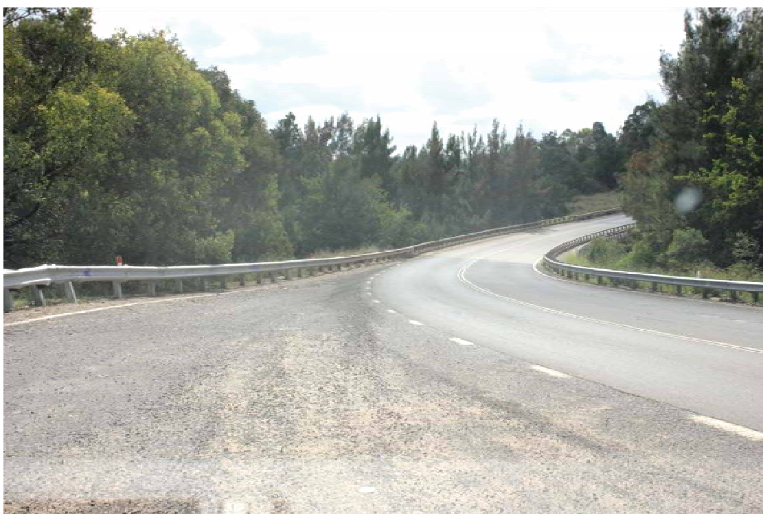
Photograph 6.5 Menangle Road 1 km north of Station Street looking north
