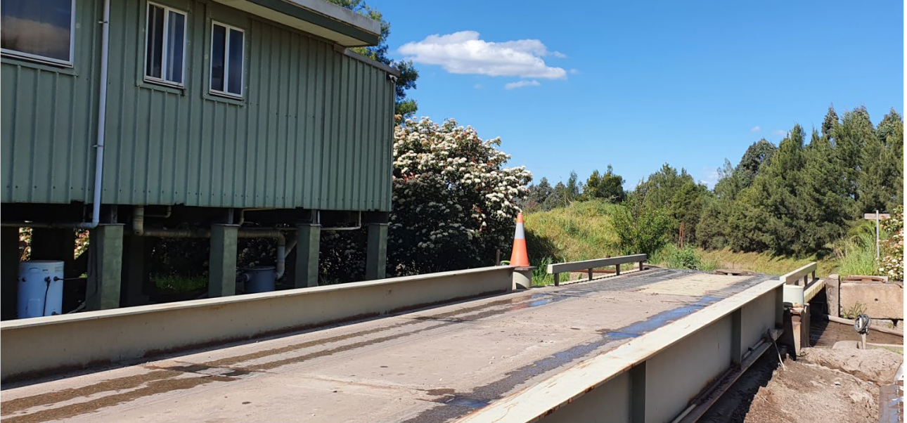
Plate 4.3 Wheel wash bay at the beginning of the weighbridge
