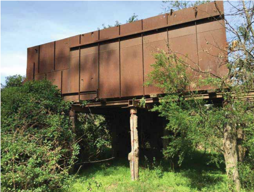
Plate 4.2 Loading bin, west elevation. The middle strut has notches cut into the sides possibly to accommodate cross beams.
