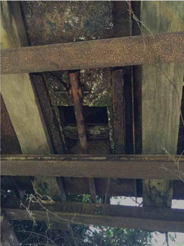
Plate 4.3 Underside of loading bin showing one of the eight sliding doors.
