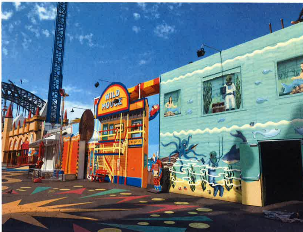
Figure 6: Current view of eastern façade along the Midway toward entrance (Source: Department's photograph)
