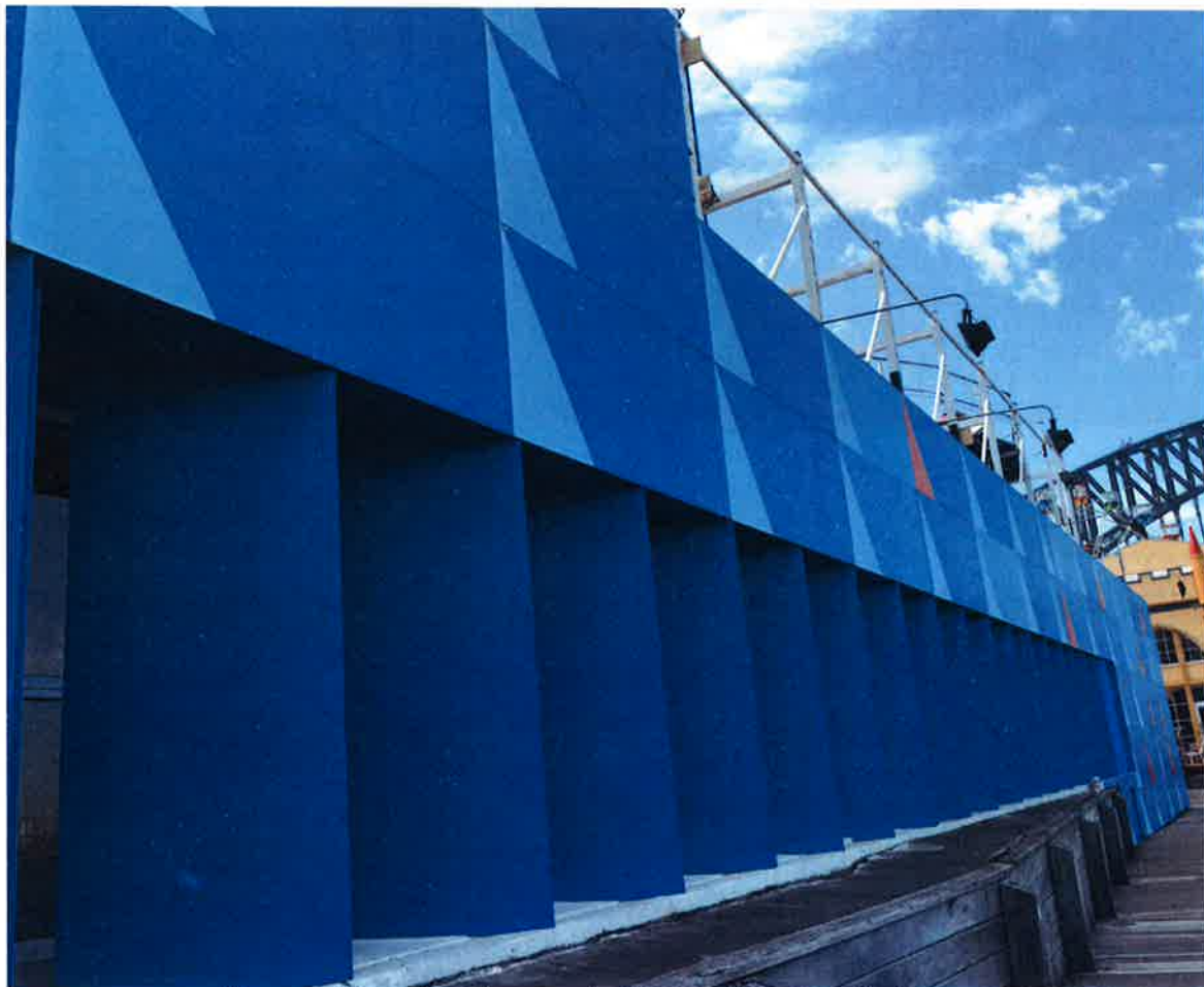
Figure 9: Current western façade (Source: Department’s photograph)
