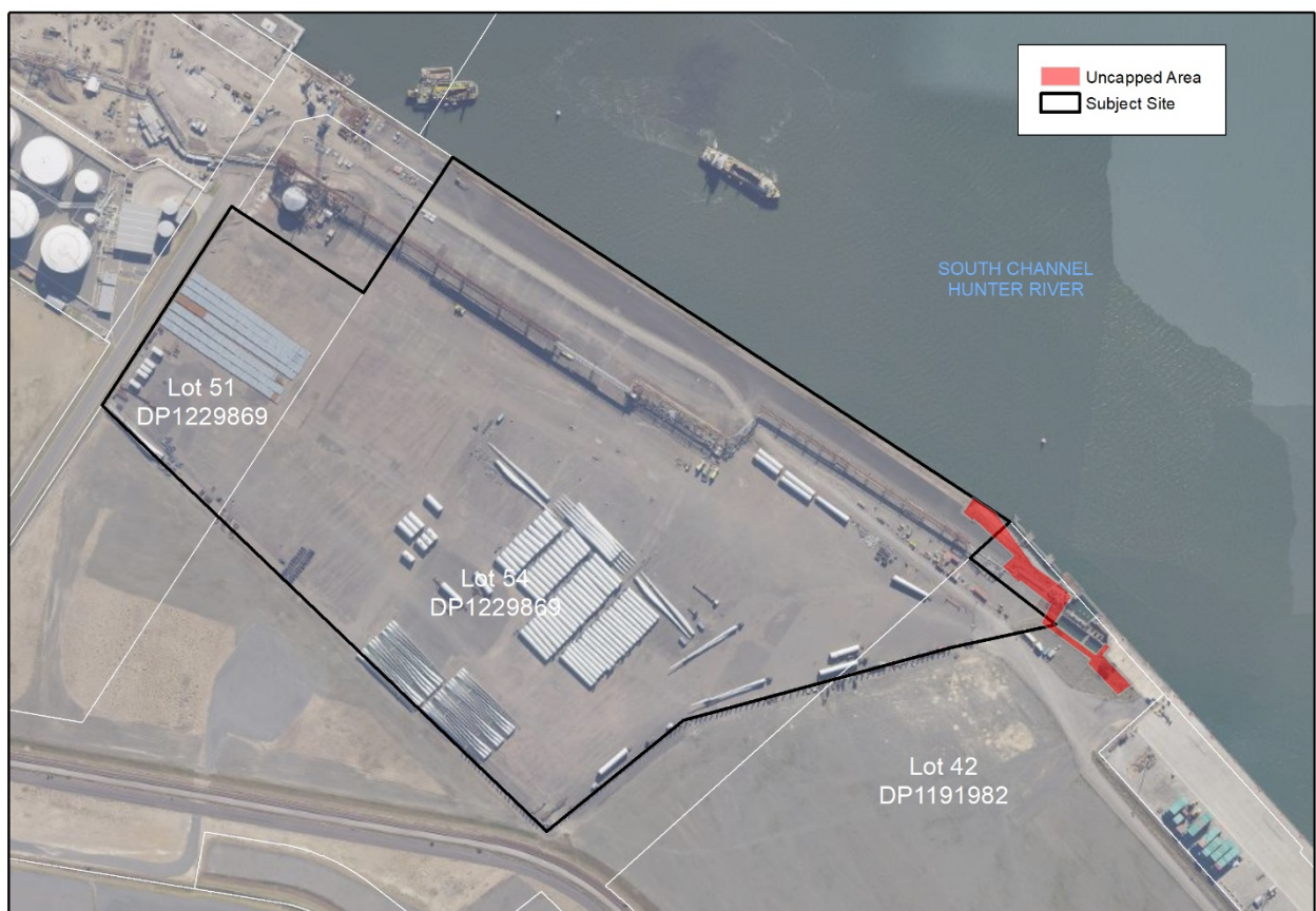
Figure 3: Uncapped land area within subject site
