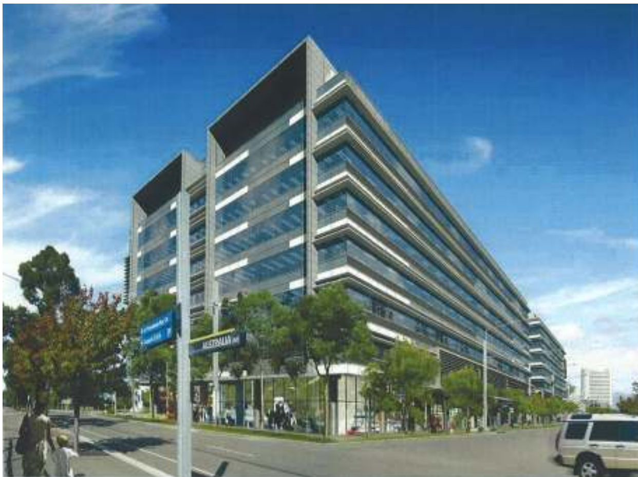
Figure 4: View of Building 7 looking west across Australia Avenue. Note the location of the reconfigured retail components at ground floor for both building 6 and 7.
