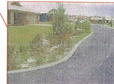
Typical WSUD bioretention swale treatment along a minor local road.
