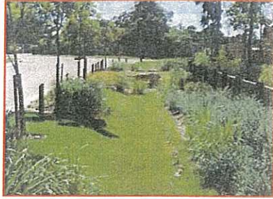
Typical WSUD vegetated swale treatment along a minor local road.
