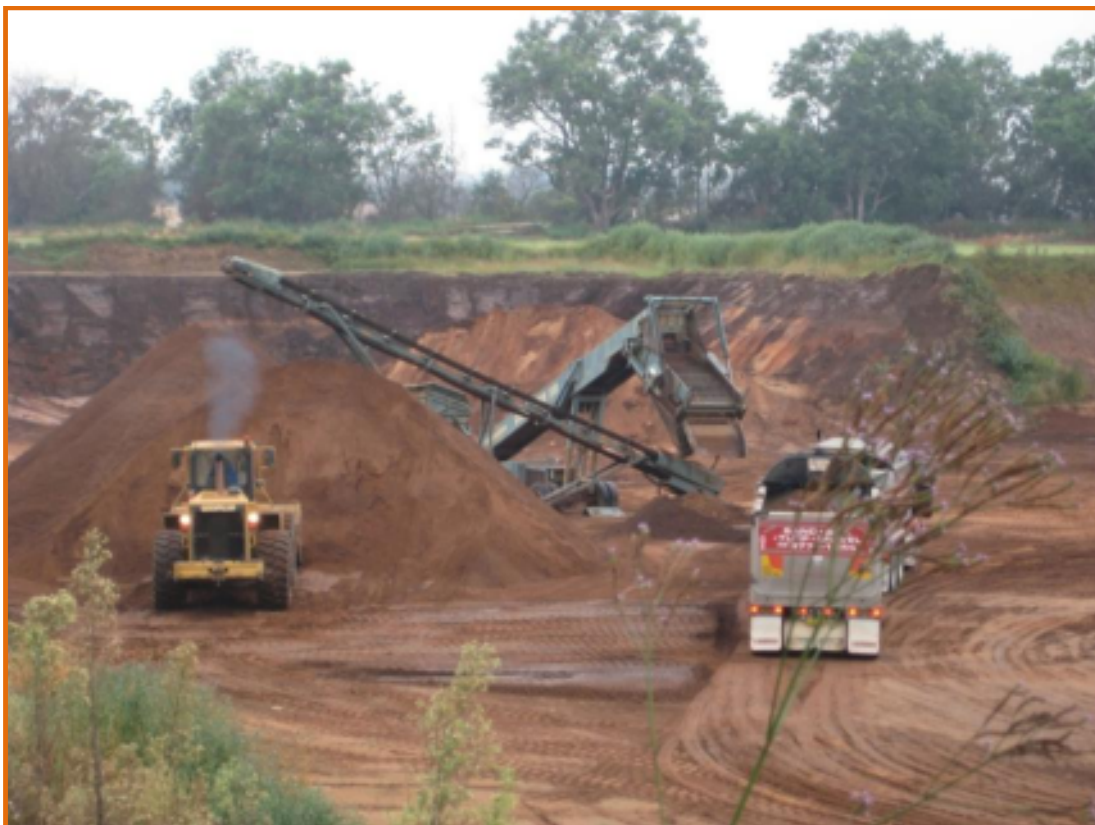
Photo 5 – Photograph shows the existing sand extraction operations using large front end loaders, particle size screens and articulated highway trucks for removing finished product. Note height of temporary batters around sand extraction typically 6 to 7 metres.
