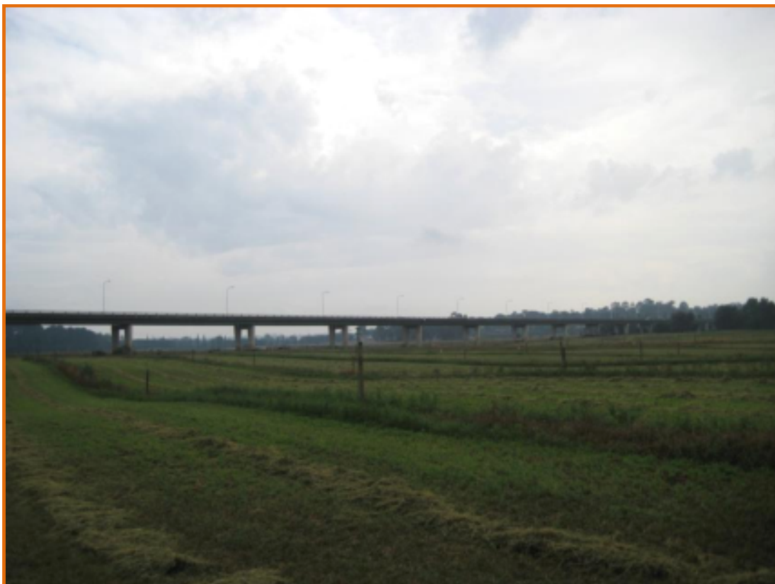
Photo 2 – view from south-western corner of subject site looking north towards the elevated Camden Bypass Bridge Viaduct. Note grassed open floodplain.
