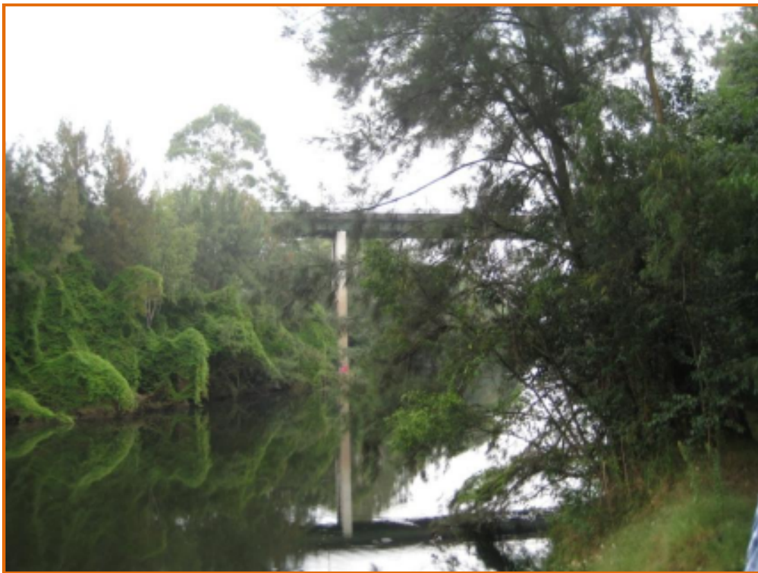
Photo 3 – view looking north towards the elevated Camden Bypass Bridge Viaduct over the Nepean River. Note height of bridge deck above river.
