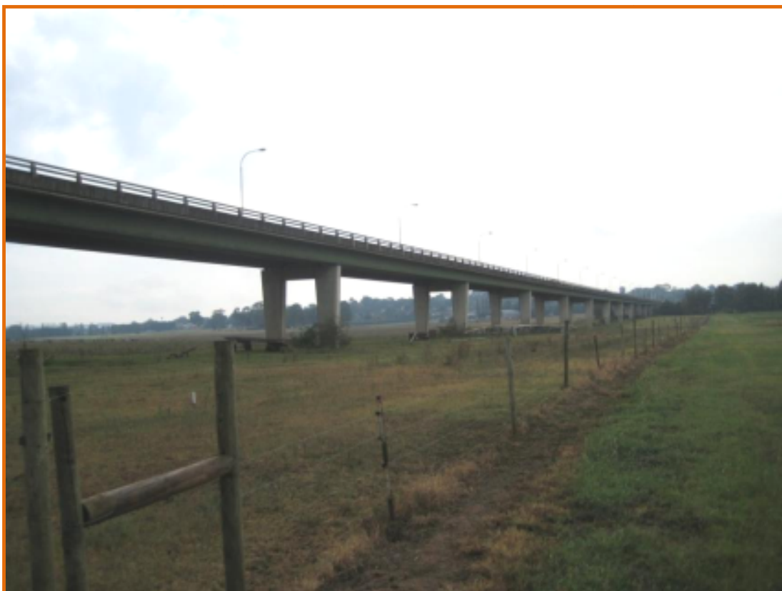
Photo 4 – view looking north towards the elevated Camden Bypass Bridge Viaduct over the Nepean River. Fence boundary in the foreground. Area between the site boundary and the bridge is characterised by grassed floodplain area.
