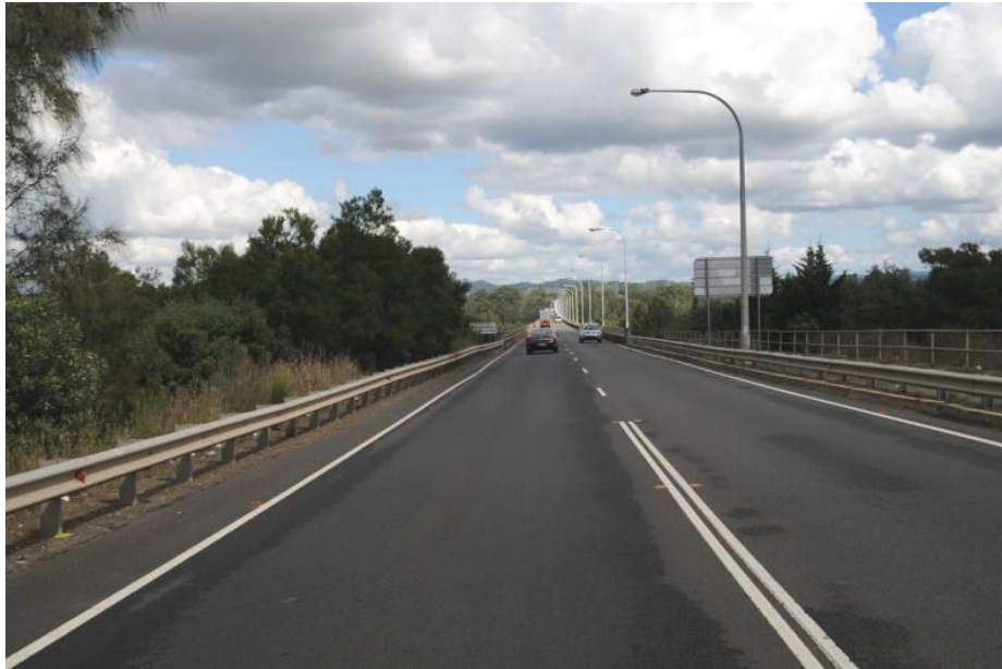
Figure 16 View west along the roadway of the Macarthur Bridge on the Camden Bypass. Once west-bound travellers reach the sign at left of centre, just past the vegetation screen, they gain views over the Nepean River floodplain, into an area currently planted with grape vines (see Fig.11 below). (Photo 6388: C Betteridge, 7 April 2004).
