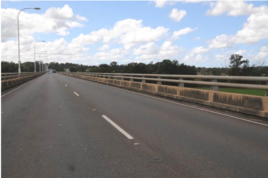
Figure 28 The view looking east along the Macarthur Bridge from a point close to the anabranck creek showing the view into the site that might be experienced by a traveller in a car or lower vehicle. (Photo 6448: Chris Betteridge, 7 April 2011).
