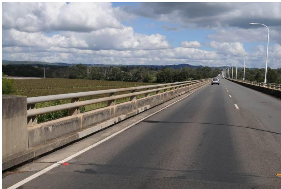
Figure 17 View west along the roadway of the Macarthur Bridge on the Camden Bypass showing the eastern part of Lot 32 currently planted with grape vines. The vegetation left of centre is along the anabranck creek. There are glimpses into the proposed extraction site through gaps in this vegetation. These glimpses could be blocked by screen plantings along the anabranck corridor. (Photo 6391: C Betteridge, 7 April 2011).
