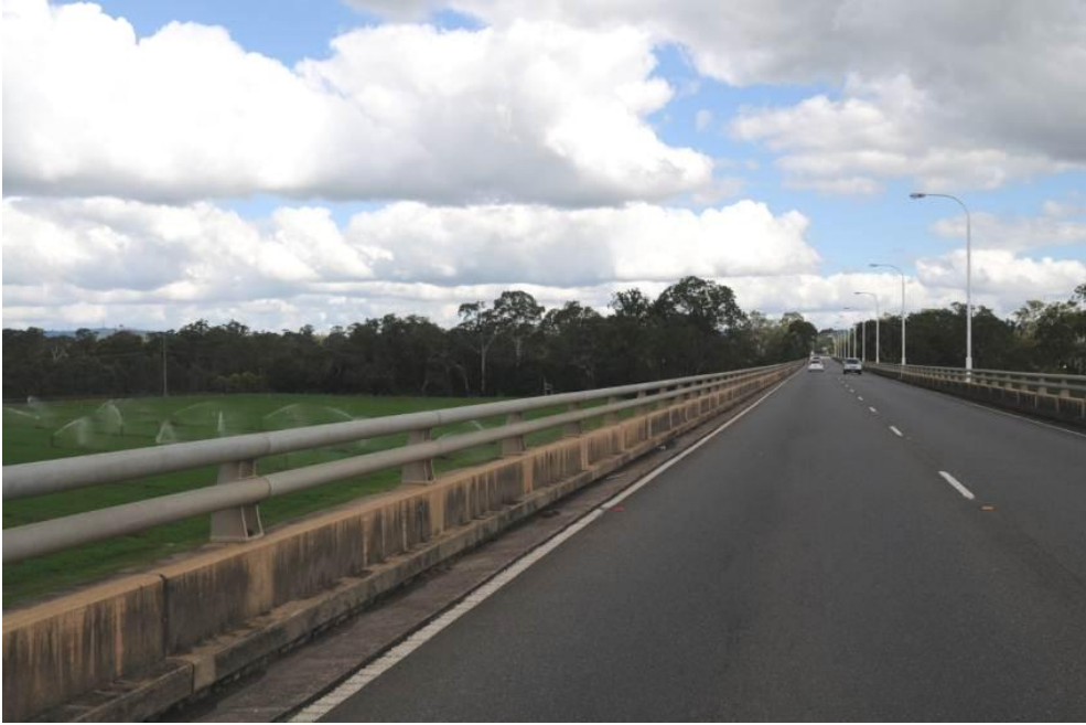
Figure 22 As for Fig.15 but showing the view from a more elevated position that might be experienced by a traveller in a truck or higher vehicle. (Photo 6418: C Betteridge, 7 April 2011).
