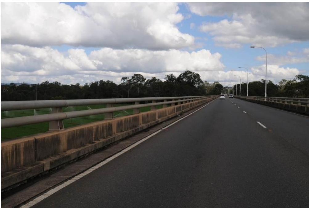
Figure 21 View from a point approximately mid-way along the proposed extraction site that might be experienced by a traveller in a car, with some restriction on the view imposed by the guard rails on the bridge. (Photo 6417: C Betteridge, 7 April 2011).
