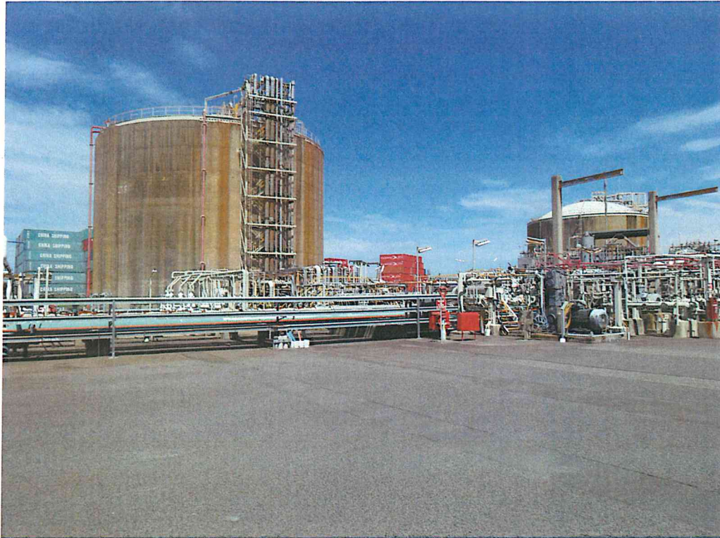
Figure 4: Photo taken on site of the propane and butane storage tanks to be demolished
