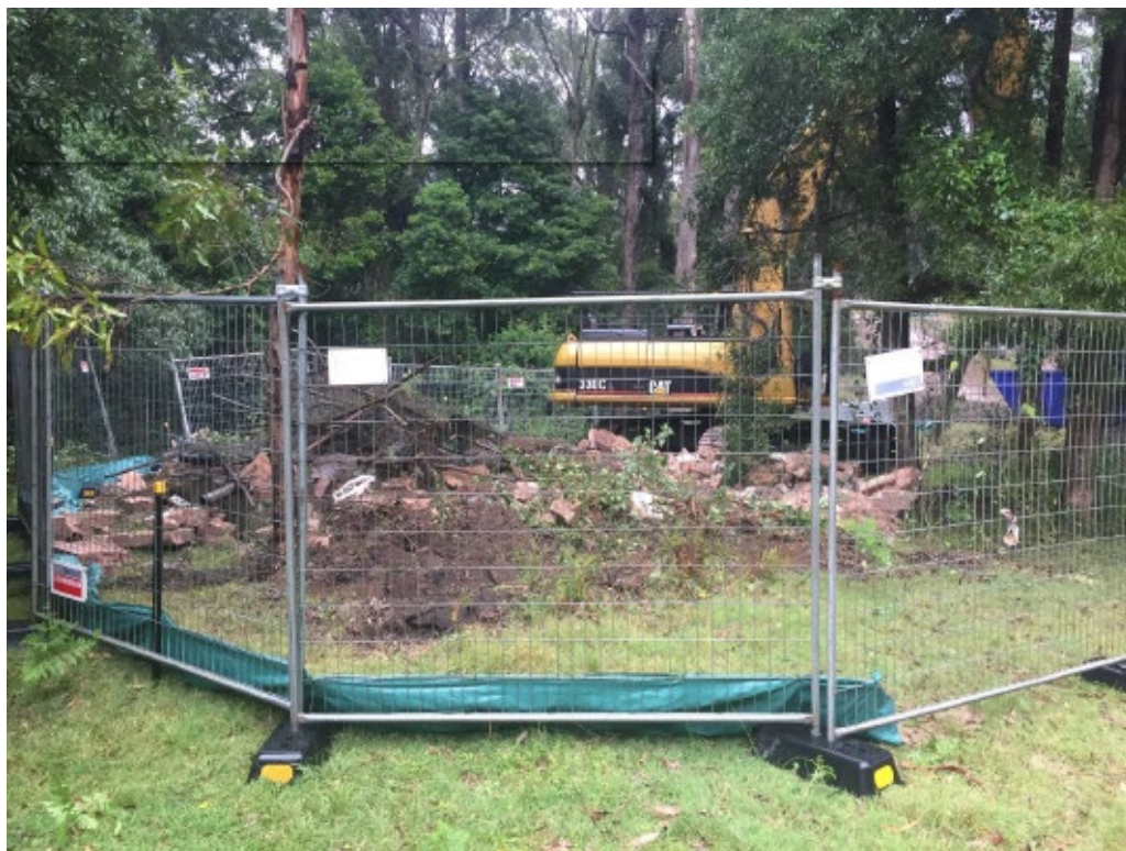
Plate 4: Demolition of O'Briens Gap Pump House
