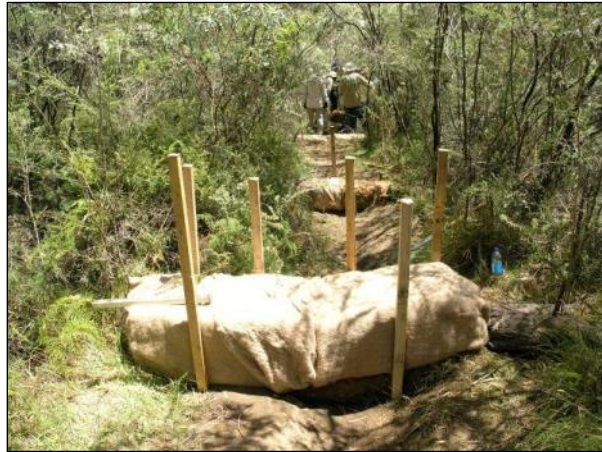
Figure 6-5 Small Coir Log Dams with Fibre Matting
