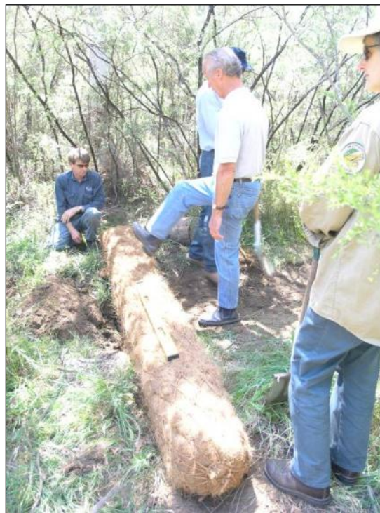
Figure 6-6 Round Coir Logs Installed to Spread Water
