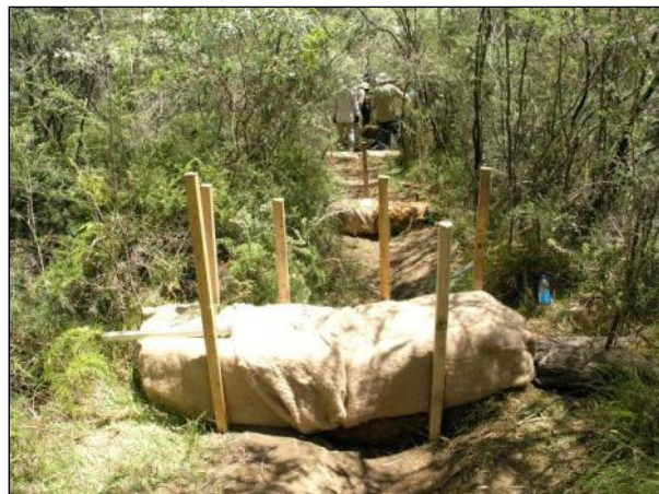
Figure 6-5 Small Coir Log Dams with Fibre Matting
