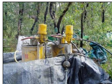
(b) Grout pump station setup
