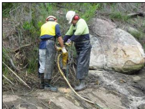
(a) Drilling into the bedrock
