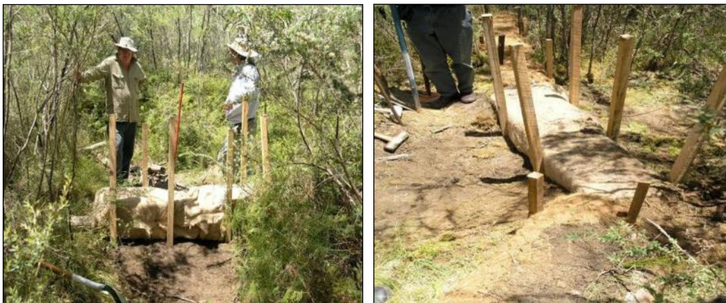
Figure 5-3 Installation of Square Coir Logs
