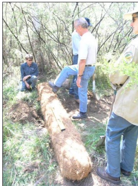
Figure 5-6 Round Coir Logs Installed to Spread Water
