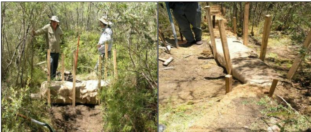
Figure 6-3 Installation of Square Coir Logs
