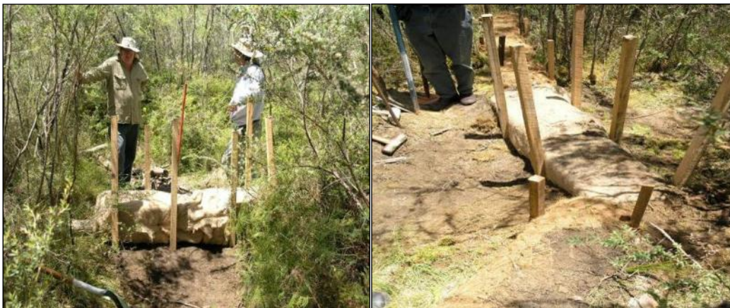
Figure 6-3 Installation of Square Coir Logs
