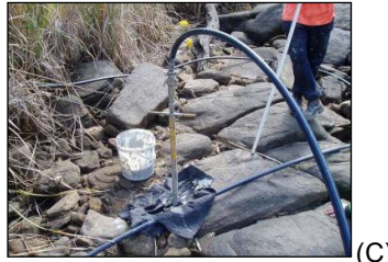
Figure 6-1: Rockbar Grouting in the Georges River - (A) Drilling into the bedrock, (B) Grout pump station setup, (C) Injecting grout into bedrock via a specially designed packer system.
