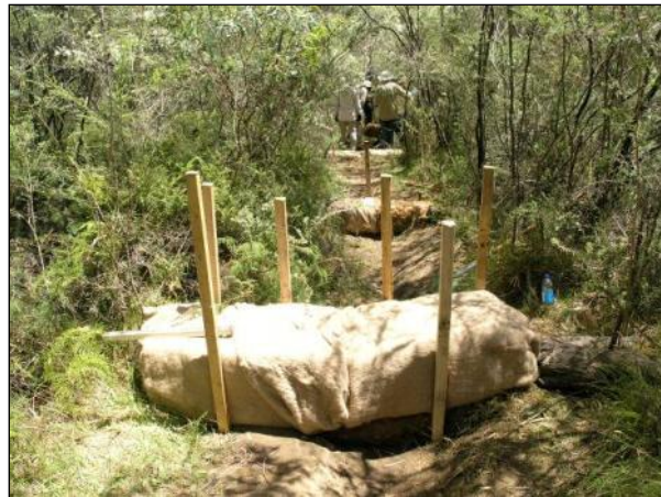
Figure 6-5 Small Coir Log Dams with Fibre Matting
