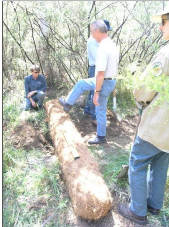
Figure 6-6 Round Coir Logs Installed to Spread Water
