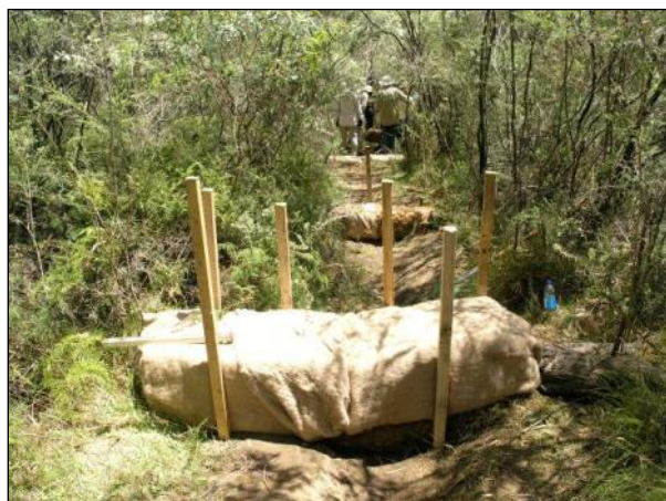
Figure 5-5 Small Coir Log Dams with Fibre Matting
