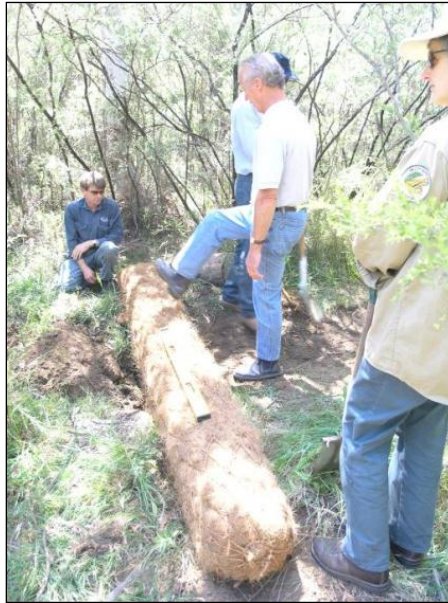
Figure 5-6 Round Coir Logs Installed to Spread Water
