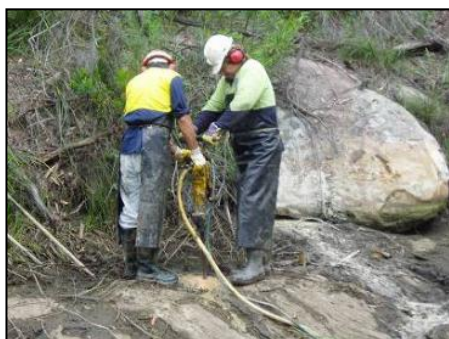
(a) Drilling into the bedrock
