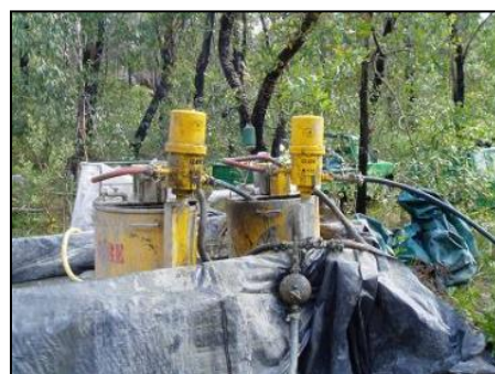
(b) Grout pump station setup
