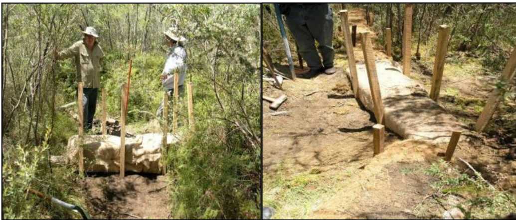
Figure 6-3 Installation of Square Coir Logs
