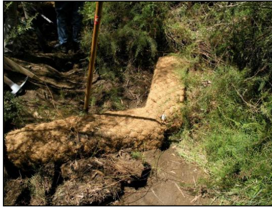
Figure 6-2 Square Coir Logs for Knick Point Control
