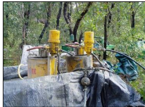
(b) Grout pump station setup
