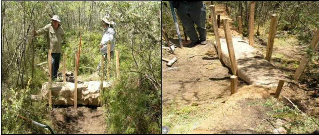
Figure 6-3 Installation of Square Coir Logs
