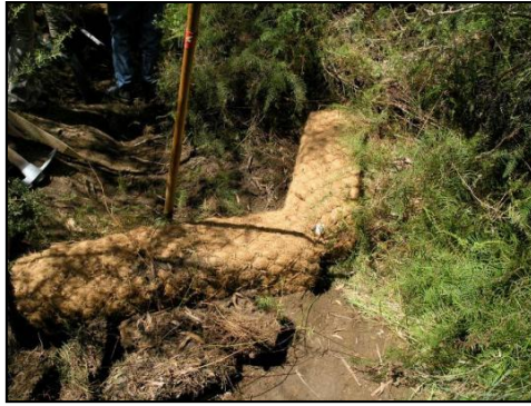
Figure 5-2 Square Coir Logs for Knick Point Control
