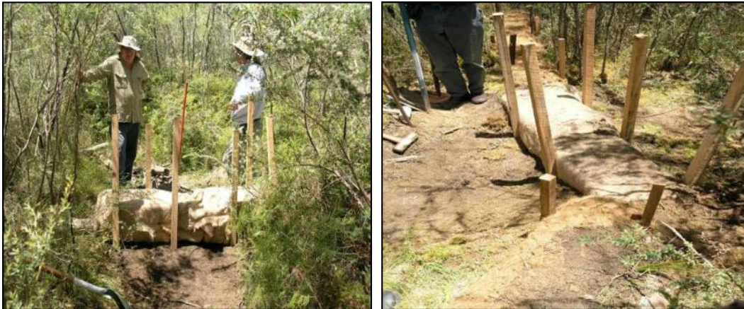
Figure 5-3 Installation of Square Coir Logs
