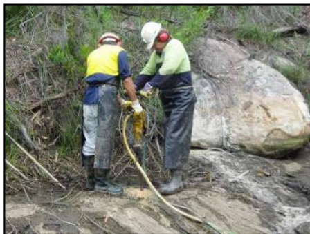
(a) Drilling into the bedrock
