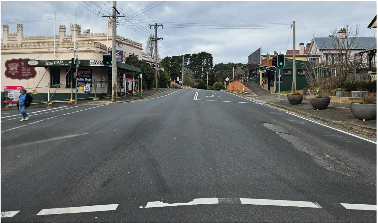
Photograph 2.5 Great Western Highway, view in south-east direction near Station Street
