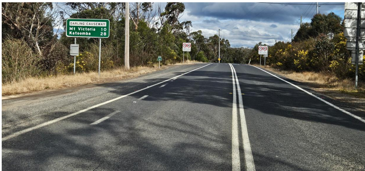
Photograph 2.3 Darling Causeway, southbound view from Bells Line of Road intersection
