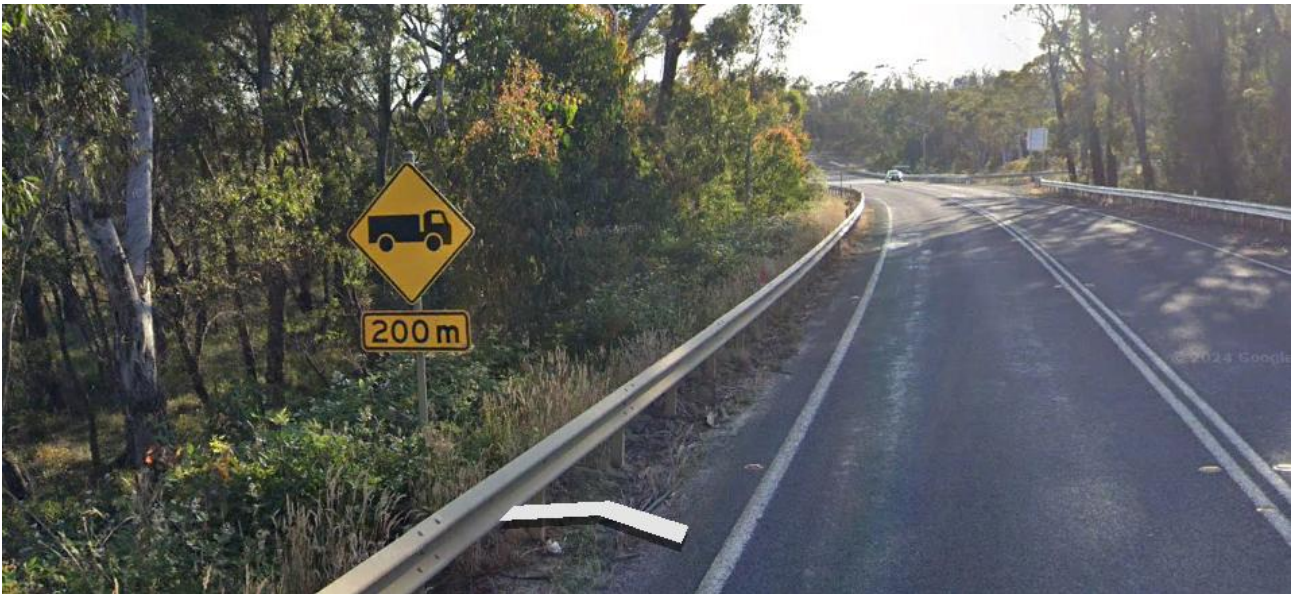
Photograph 4.3 Trucks crossing or entering sign (W5-22) on Chifley Road eastbound approach to Clarence Colliery Road
