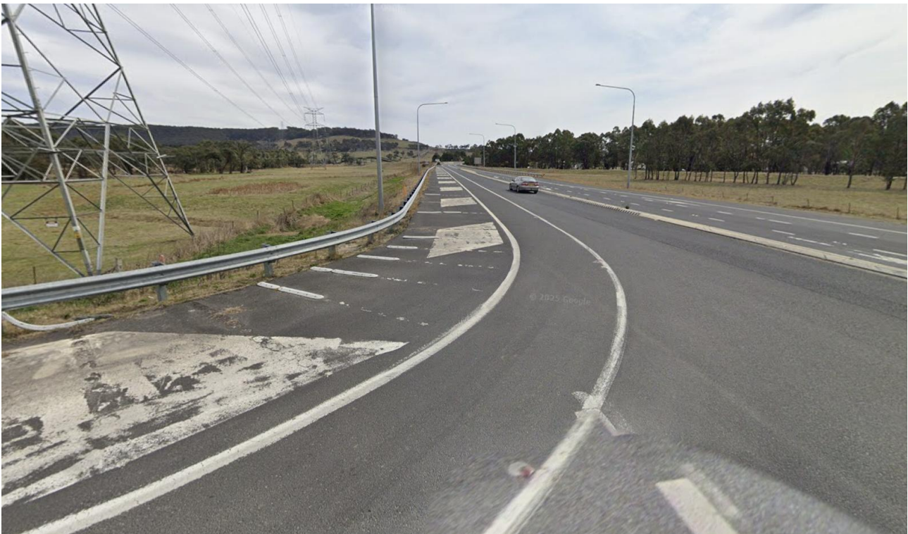
Photograph 4.6 View to the left from Main Street to Castlereagh Highway
