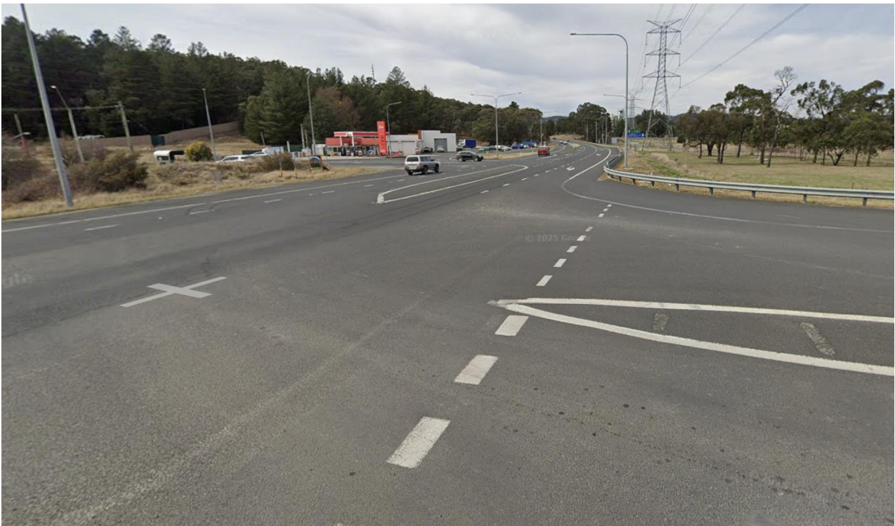
Figure 4.5 Sight distance to the left from Main Street to Castlereagh Highway (260 m)
