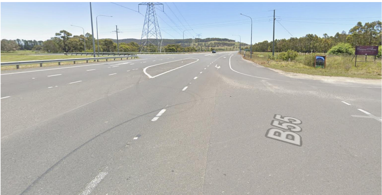
Figure 4.7 Sight distance to the left from Wolgan Road to Castlereagh Highway (235 m)
