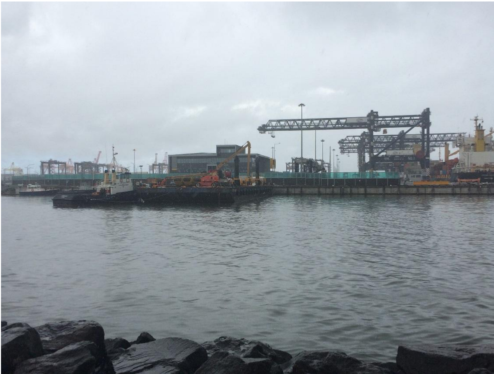
Plate 1: View of site from Boat Ramp area, with SICTL's stevedores in the background
