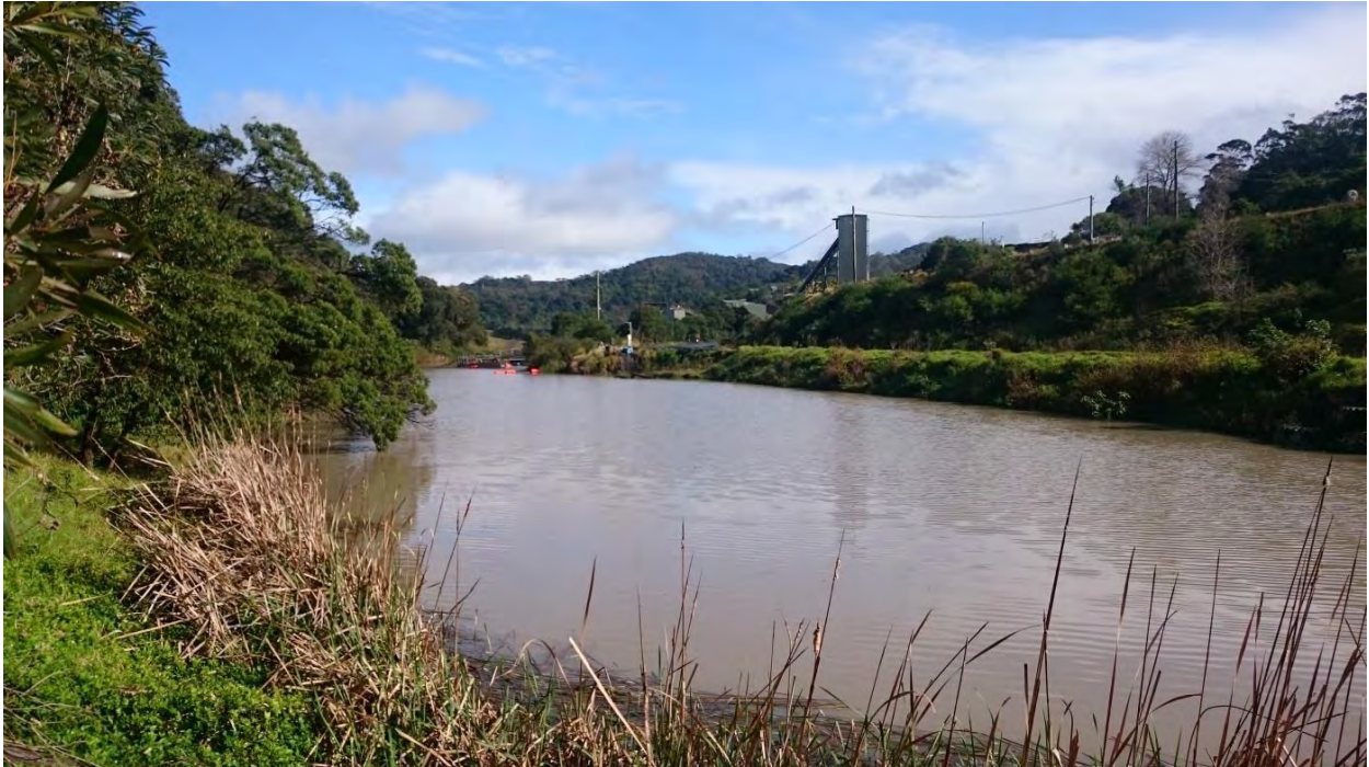
Photo 4 – shows the Lower Dam (looking west)
