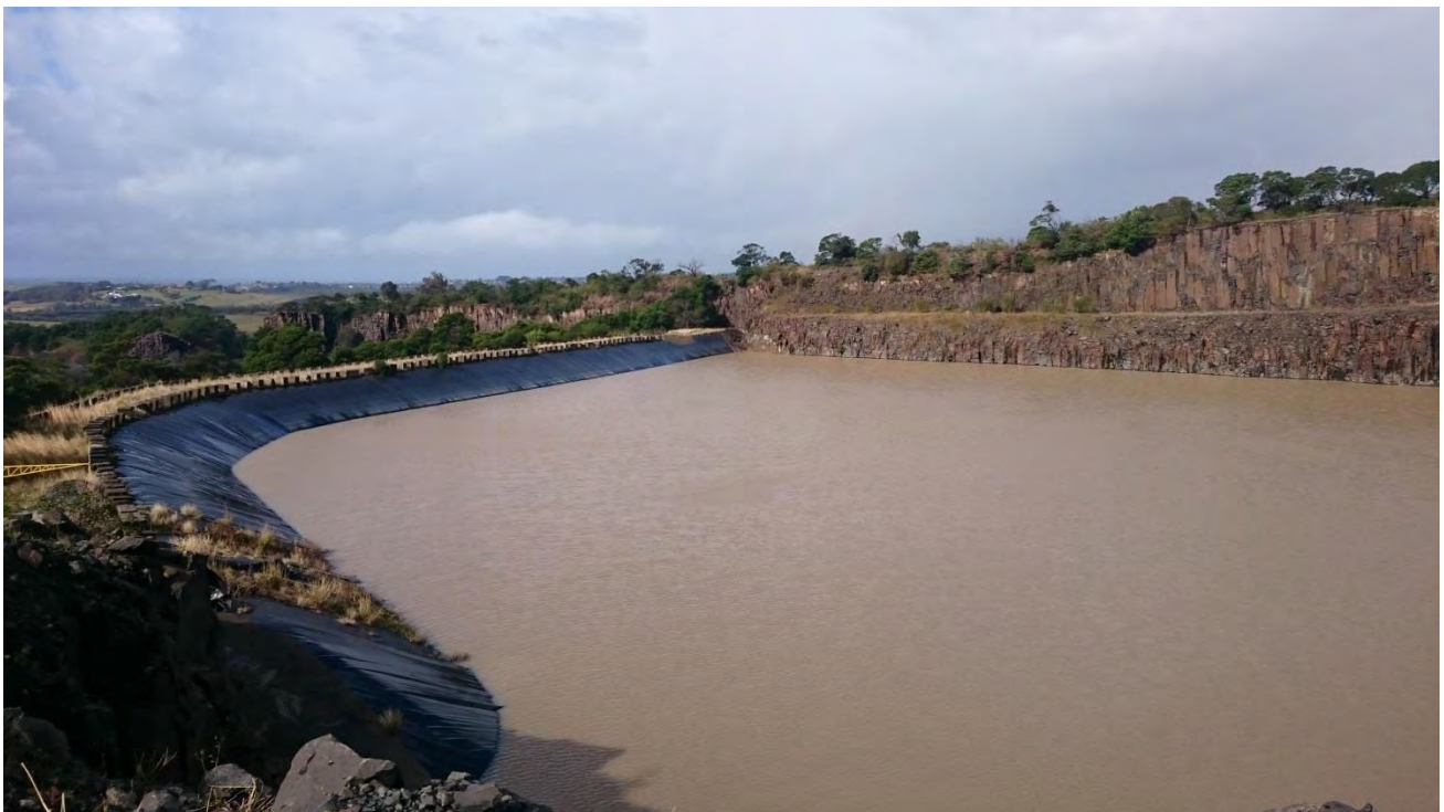
Photo 5 – shows the Middle Dam (looking east)
