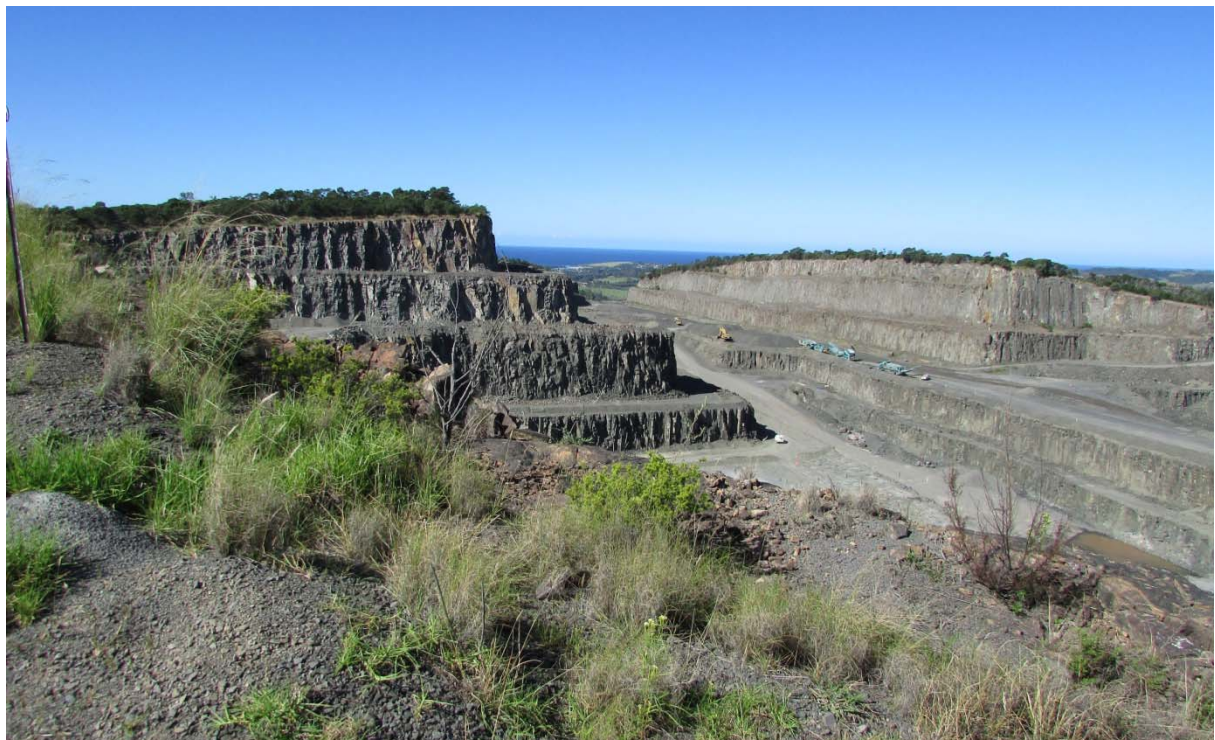
Photograph 2.1 Looking east-south-east from the north-western corner of the Croome Farm Pit towards the RailCorp extraction area
