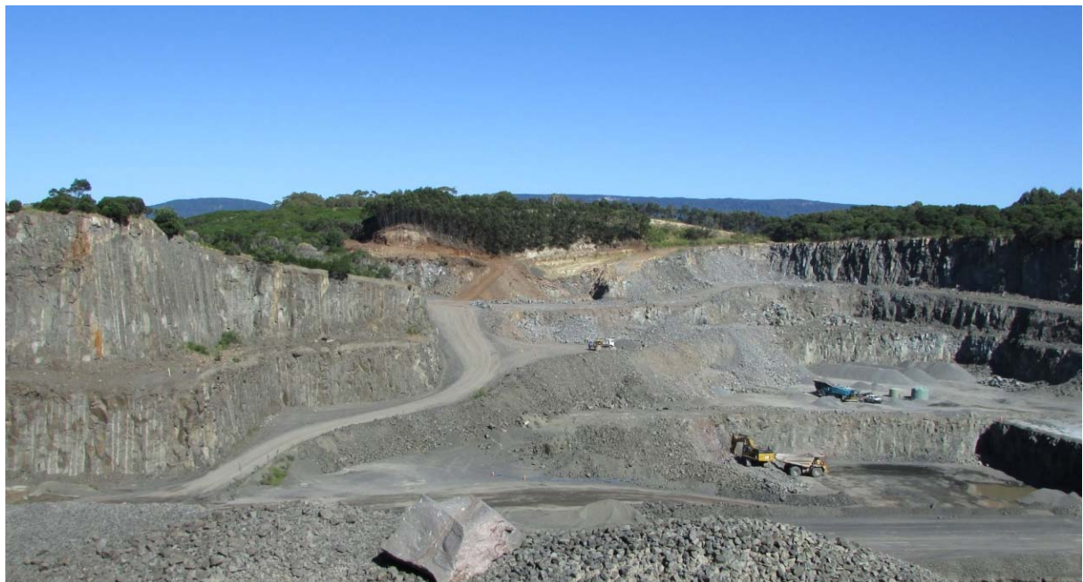
Photograph 3.1 Looking south towards overburden to be removed in the south of the Croome Farm Pit
