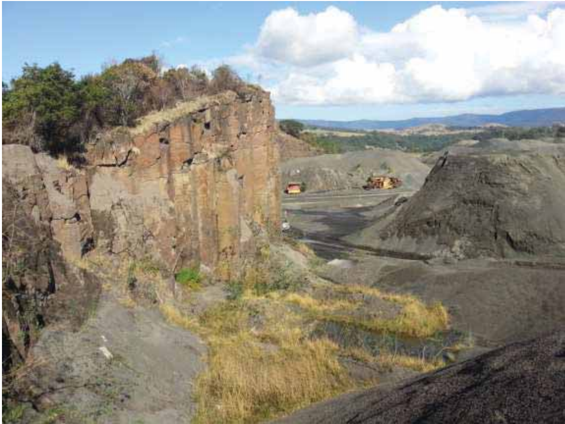
Plate 1: View of the Project Site showing the southern section of the eastern rim of the original Dunmore Quarry.
