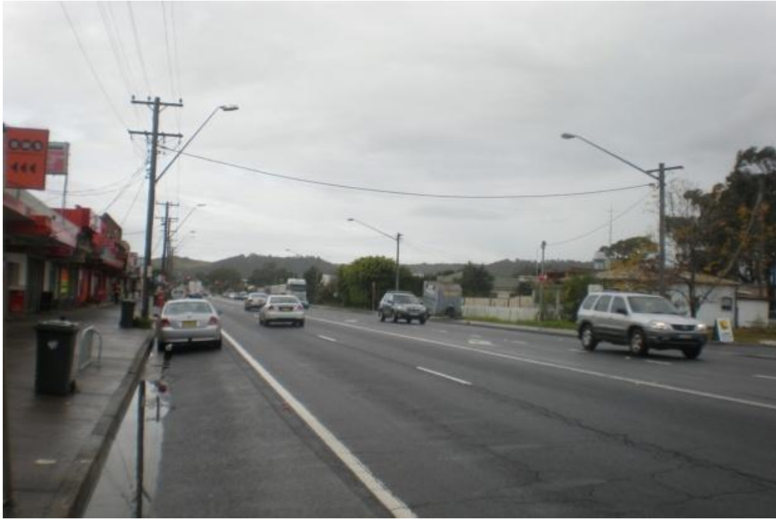
Photograph 2.1 Princes Highway at Albion Park Rail southbound
