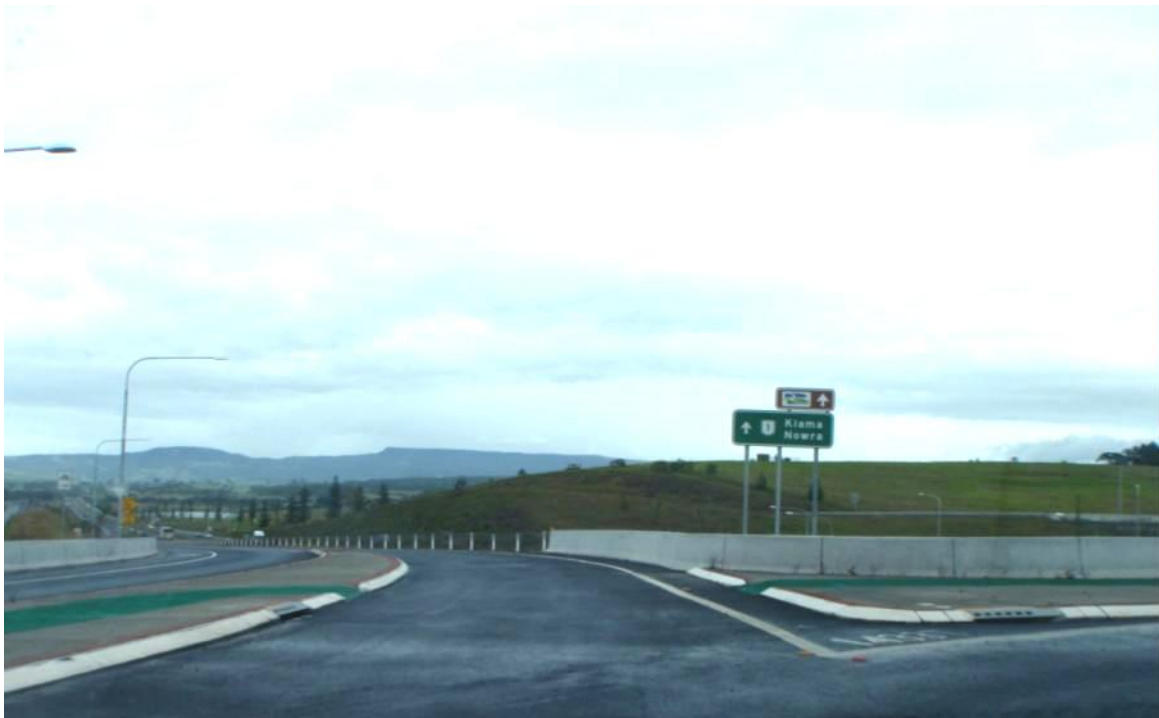
Photograph 2.6 U Turn facility for southbound site traffic at Shellharbour Road ramps
