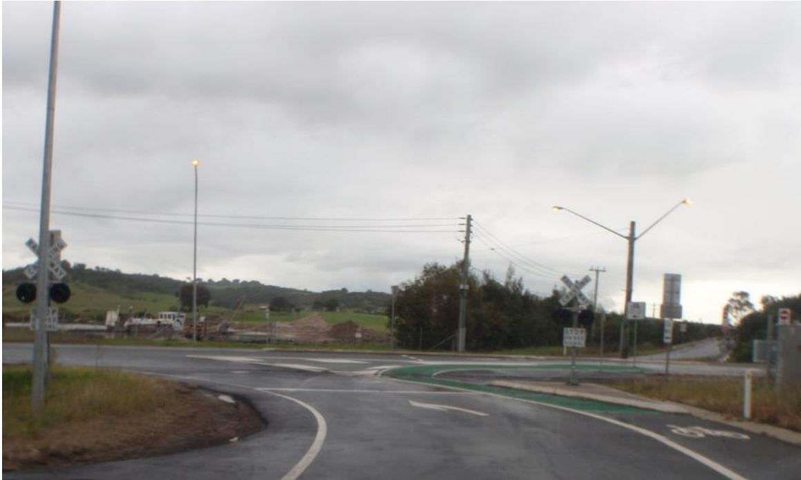
Photograph 2.7 Tabbita Road intersection with the Princes Highway ramps (west side)
