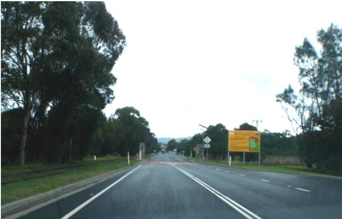
Photograph 2.8 Tabbita Road entry to the Dunmore Site- the railway siding is on the left
