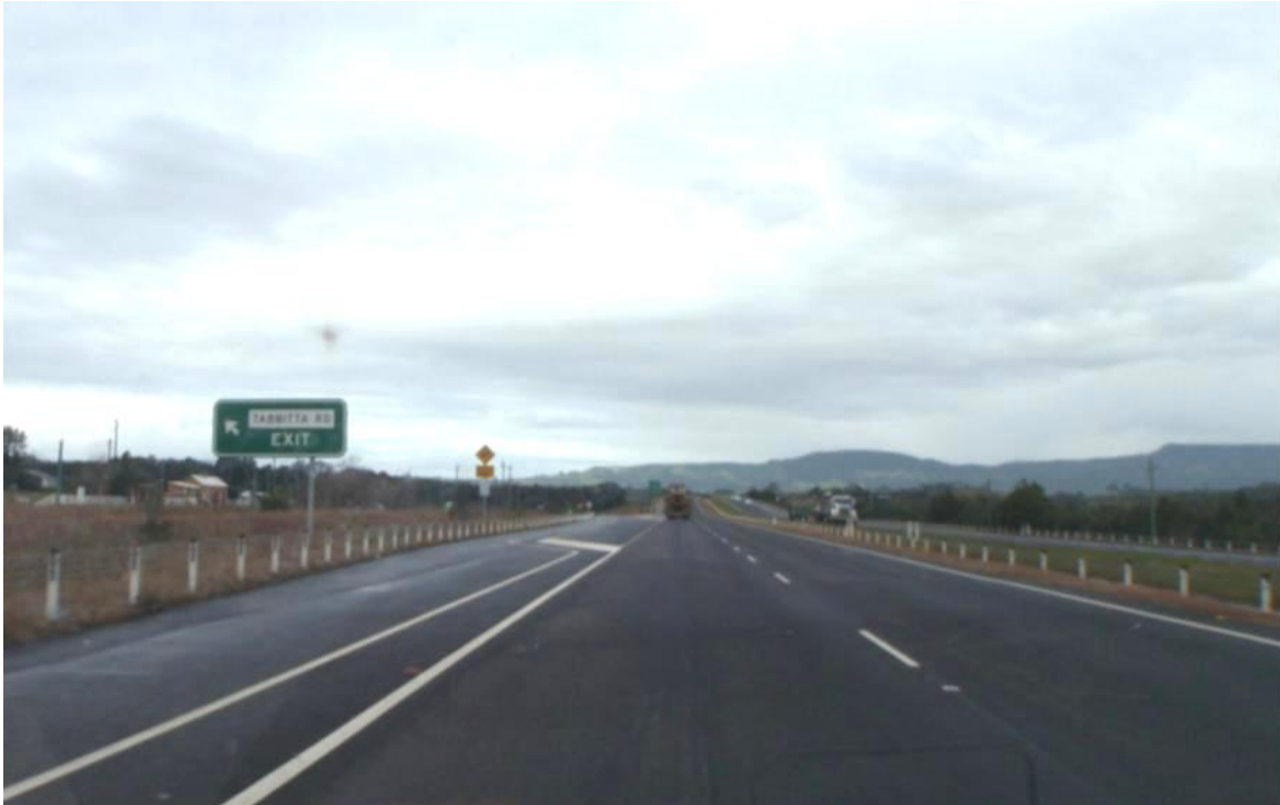
Photograph 2.3 Princes Highway exit at Tabbita Road southbound
