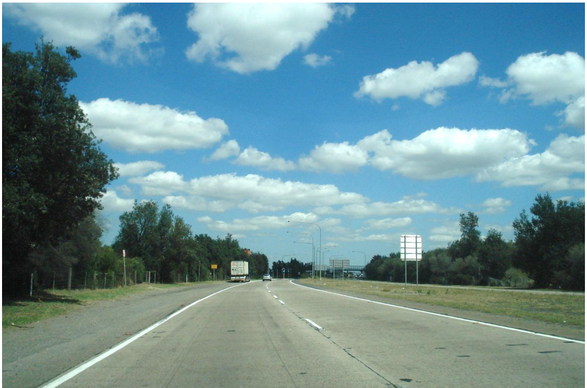
Photo 3 – Foreshore Road looking west, west of Penrhyn Road.
