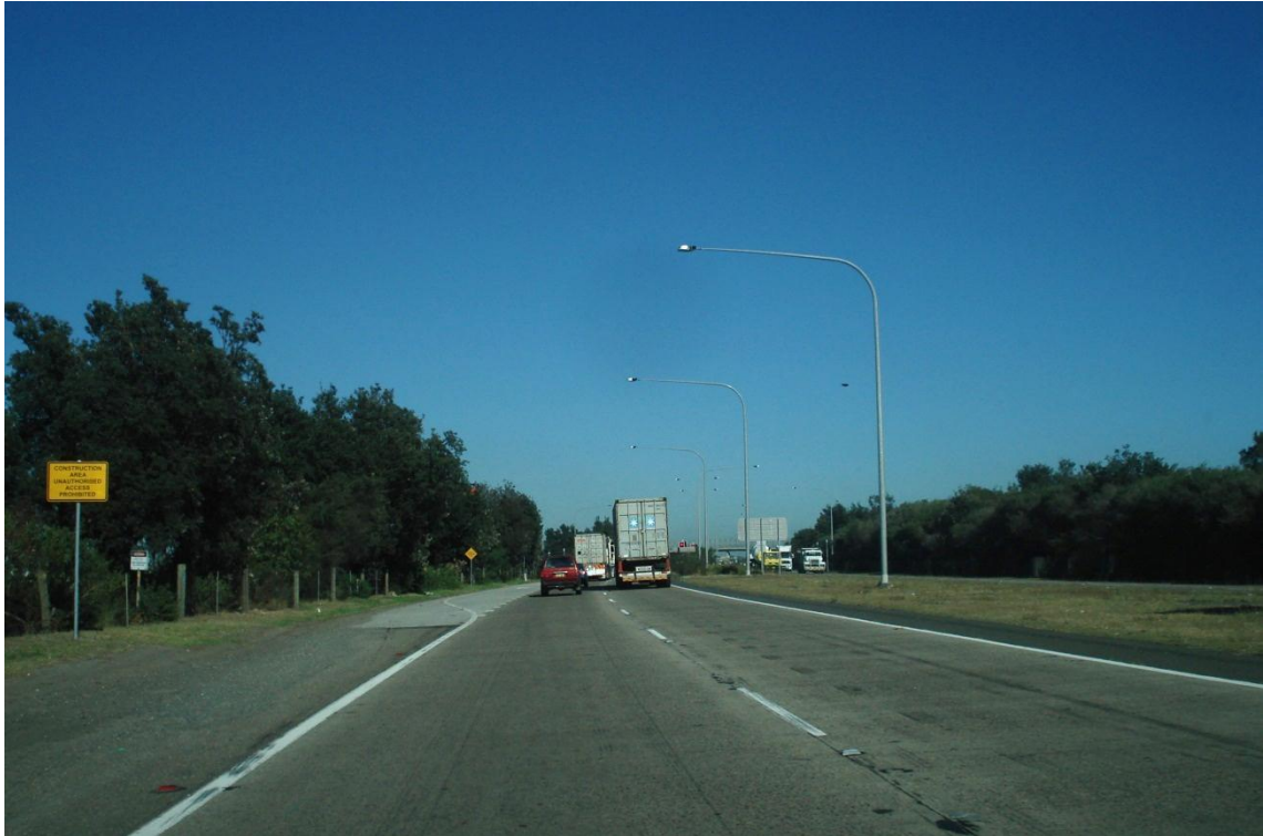
Photo 4 – Botany Road looking westbound to the east of Penrhyn Road
