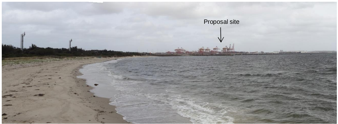
Photograph 6-4 Sensitive receptor location 4 (Mill Stream Lookout, Foreshore Beach, Botany). Existing view looking southeast from Mill Stream Lookout towards the proposal site
