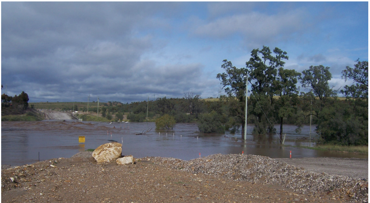
Figure B.7.8 Haul Road Bridge during June 2007 Event
