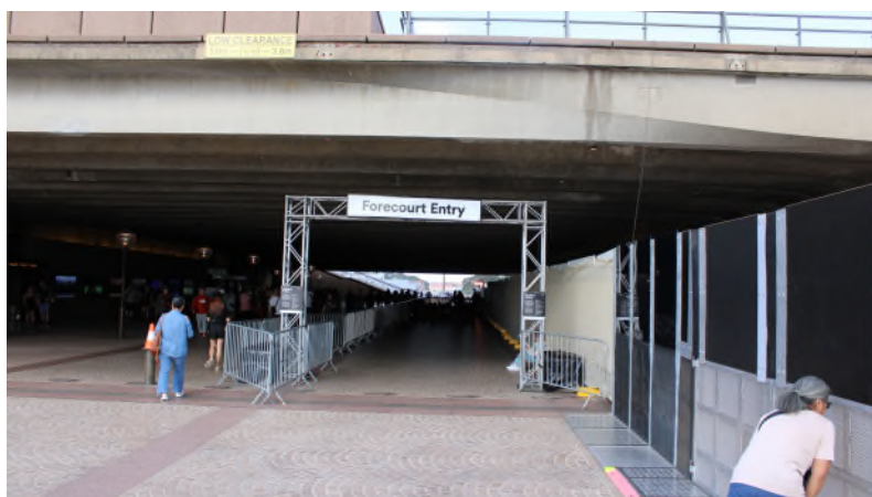
Figure 49: View to the Covered Concourse with event entry from the west. March 2025 Music series.
