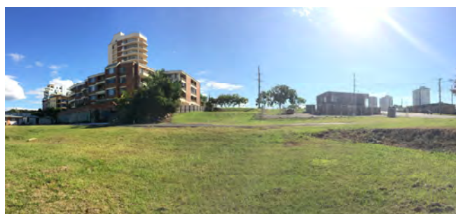
Figure 9: Existing levelled pads and batter slopes
