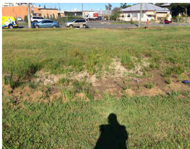
Figure 10: Existing stormwater pit
