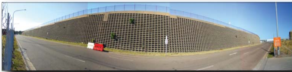
Figure 2 - Prince of Wales Drive revetment wall opposite the site
