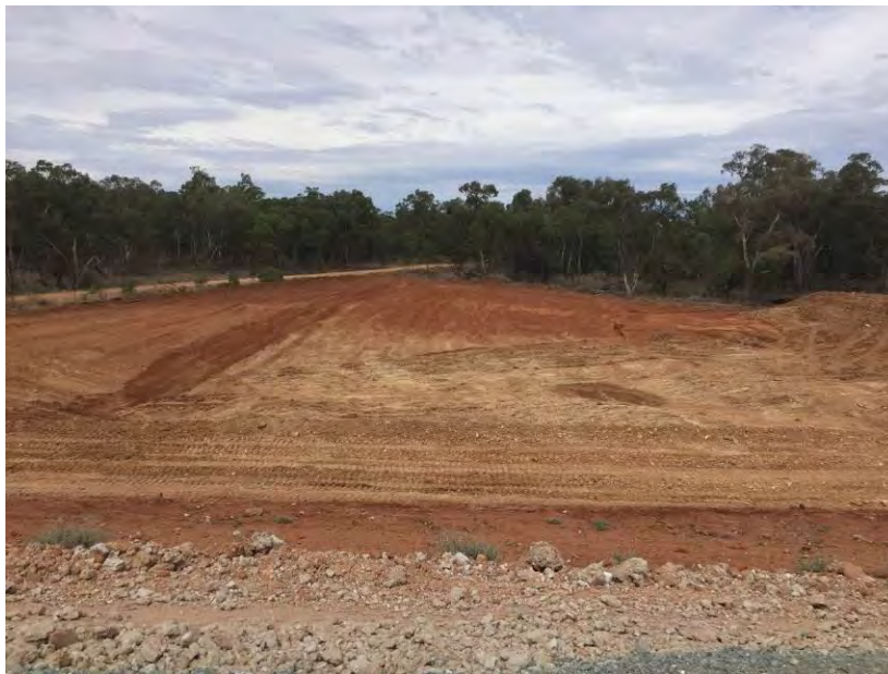
Plate 2 - Dam Storage Excavated
