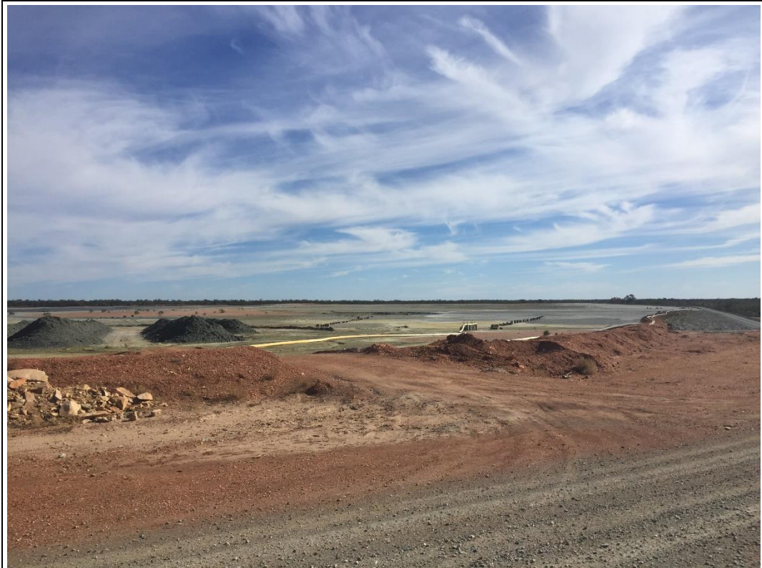
Plate 1 Example of Tailings Storage Facility Access Point
