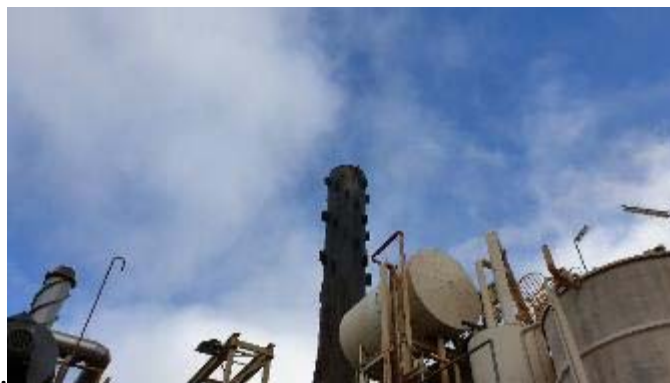
Photo 4: Boiler emissions opacity monitor reading 30-50%; minimal smoke evidence at 34.1%.
