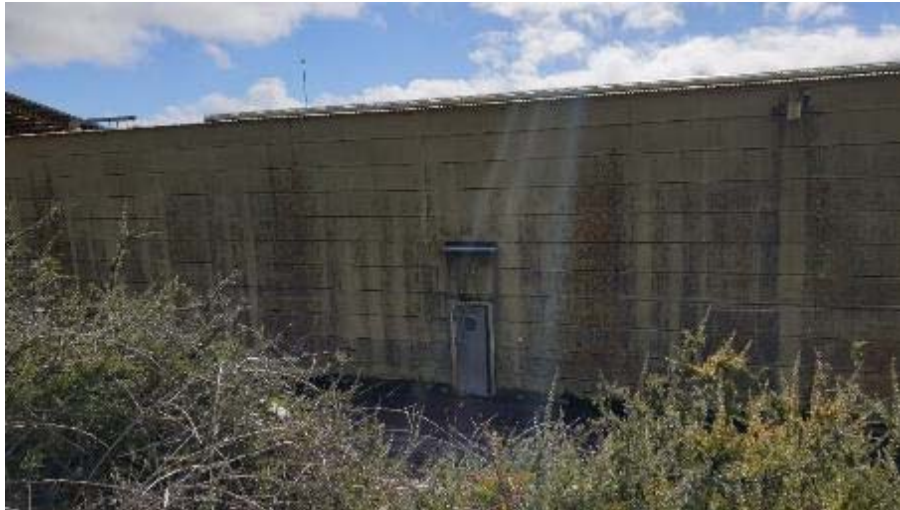
Photo 6: Southern door ajar represents a pathway for noise escape during night.
