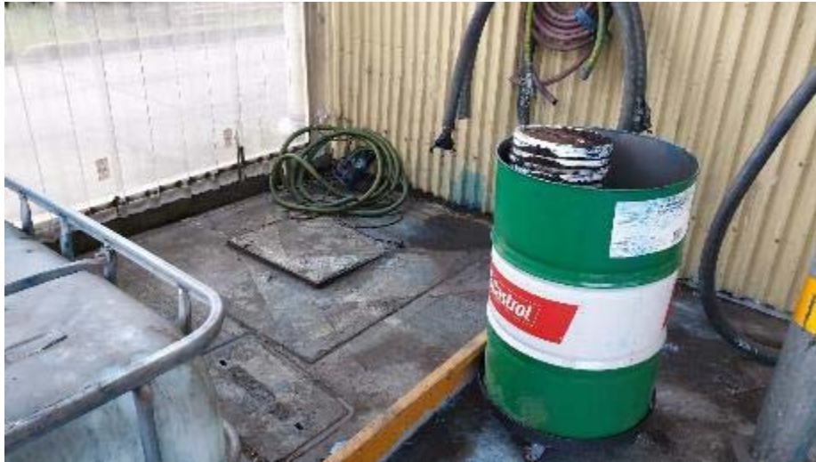
Photo 9: Hose hook up area is outside bund and can drain to below ground services.
