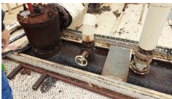
Photo 5a: Boiler top not insulated leading to inefficiencies & additional fuel requirements. Rec. Insulate the boiler top and valve stems.
