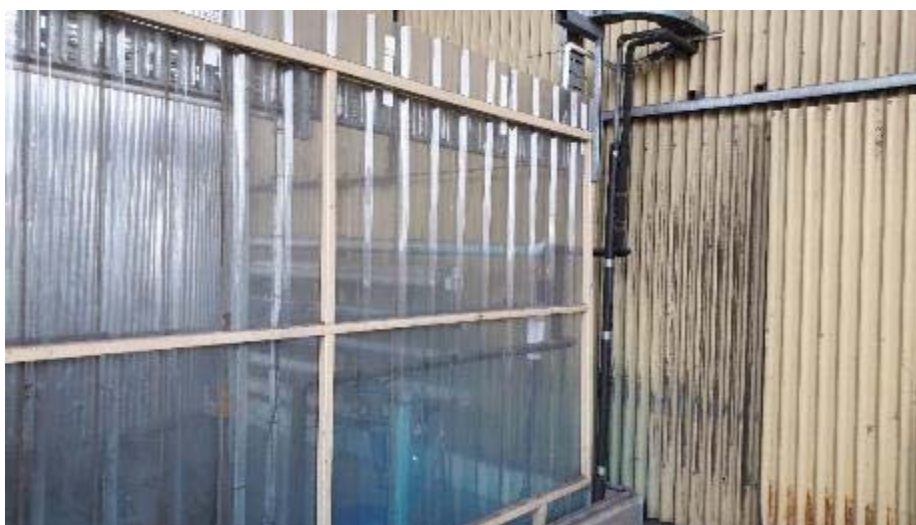
Photo 8: Pipe identification not present and pipes extend outside bund.
