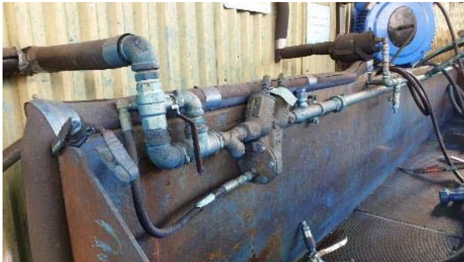
Photo 10: Backflow prevention may not be on in-feed line. Rec. Check location of backflow control.
