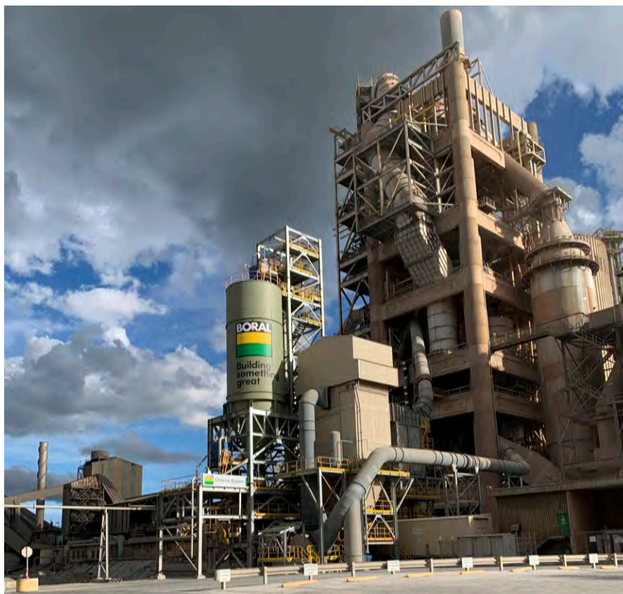
Figure 1.1: View of the CBP from the north-west, with the Kiln 6 Preheater tower behind
