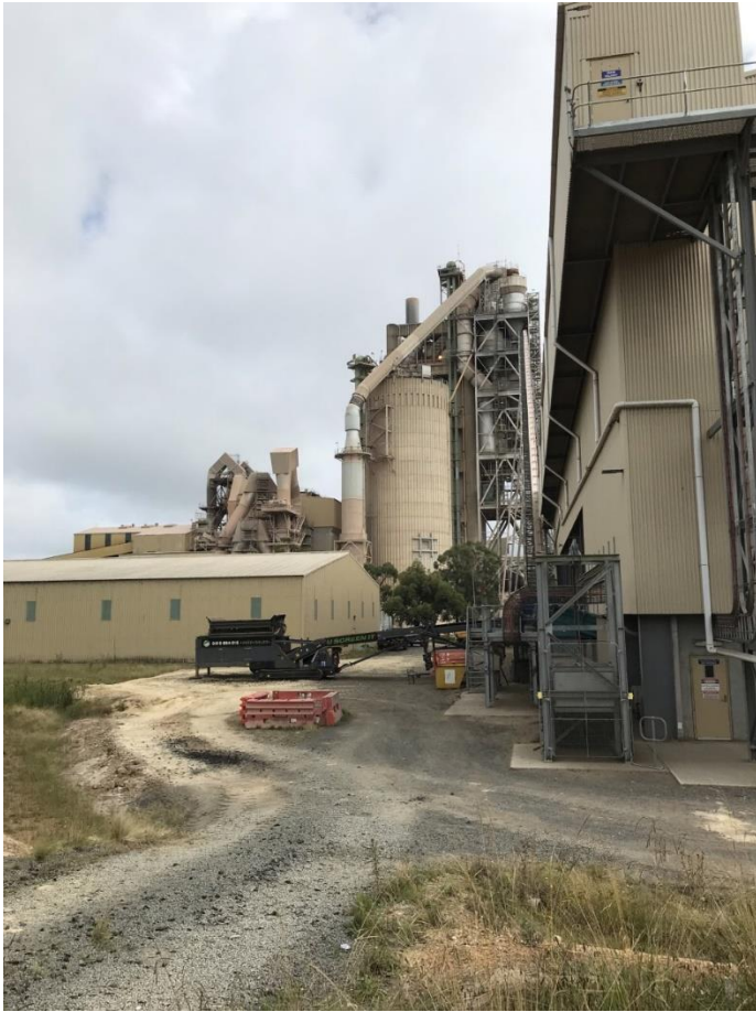
Photo 4: Feed location onto SWDF conveyor into calciner.
