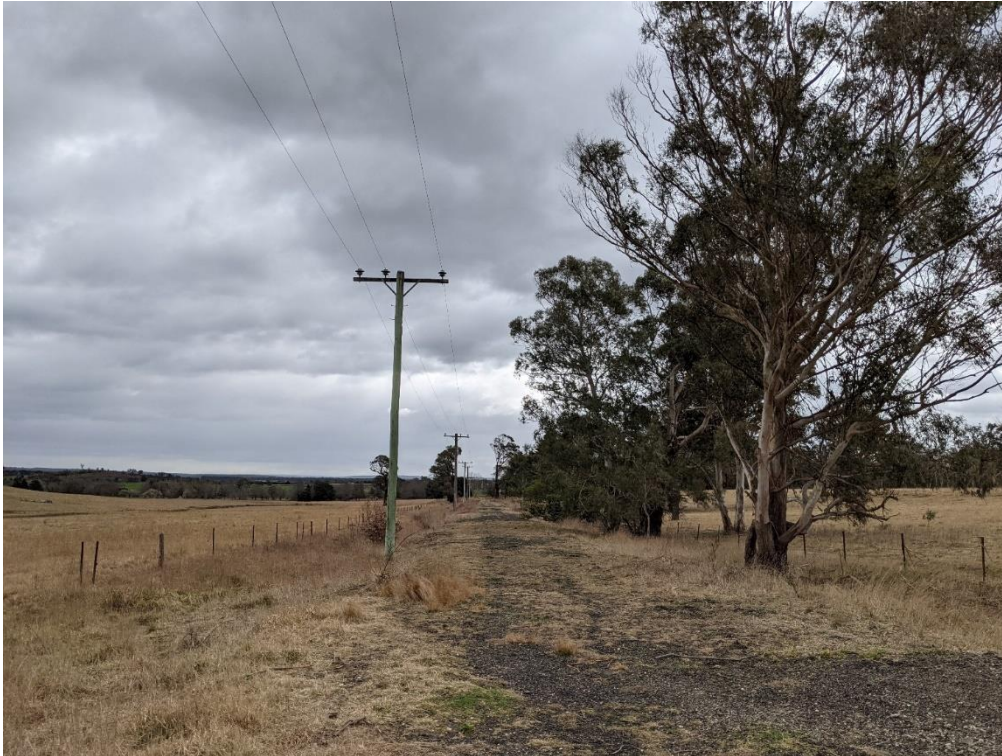
Photo 1 Existing powerline easement for original proposed alignment.
