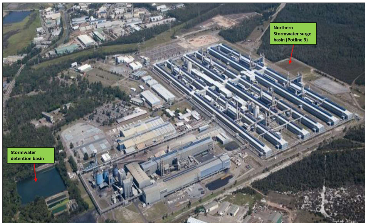
Figure 5: Site stormwater surge basin and stormwater detention pond
