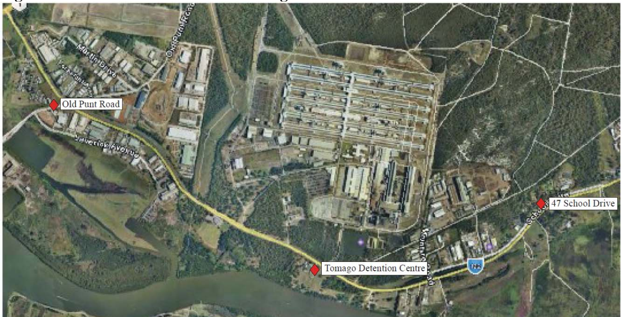
Figure 10: Environment Noise Monitoring Sites
