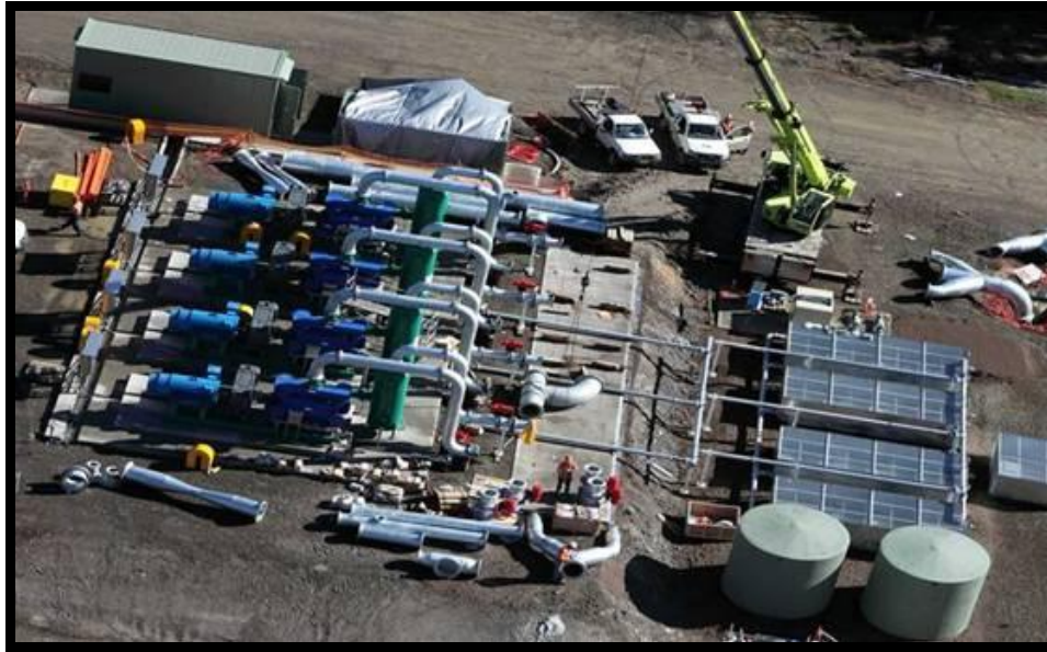
Plate 8 – Goaf Gas Drainage Plant at BFS Underground Mine under construction.
