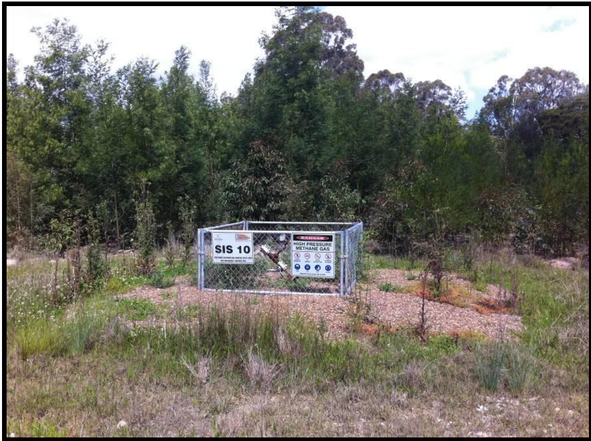
Plate 4 - SIS well head following drilling and pad rehabilitation.
