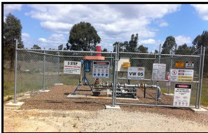
Plate 1 – Existing Vertical Well above a longwall panel at the BFS Underground Mine
