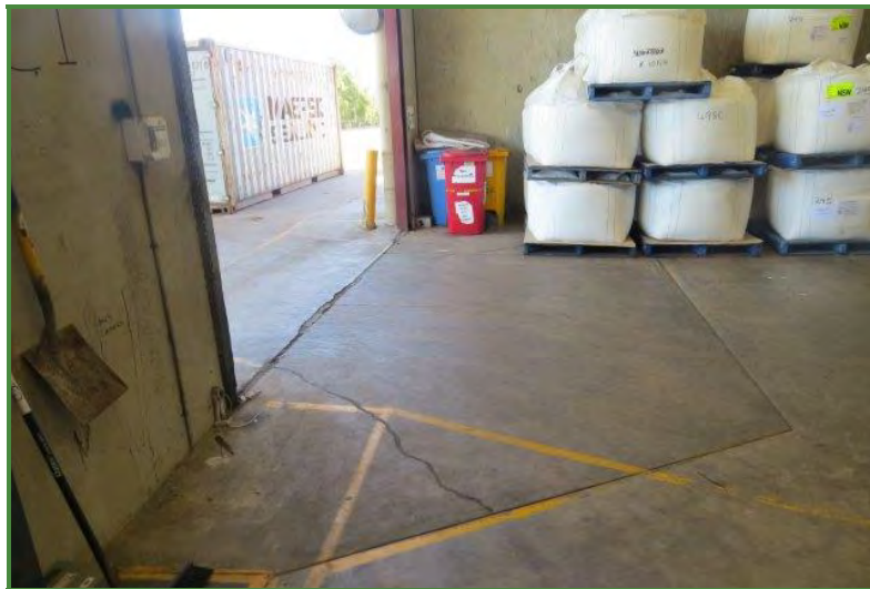
Photograph 1.5: The floor level is lowered relative to the doorways thus creating a “well”. The floor from the doorway into the lower level of the building has a gentle slope.
