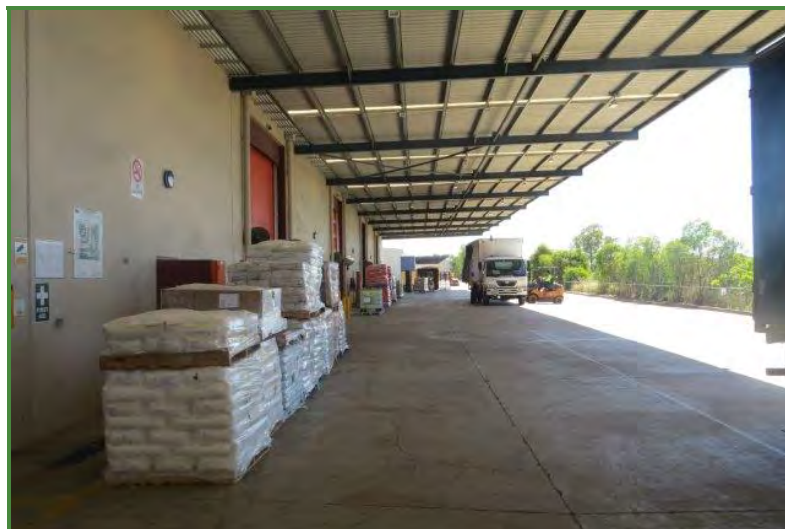
Photograph 1.9: The awning area provides all weather protection for unloading, providing a staging area for products to be loaded, and then the loading on to trucks. A small number of shipping containers are loaded for export, mainly to New Zealand.
