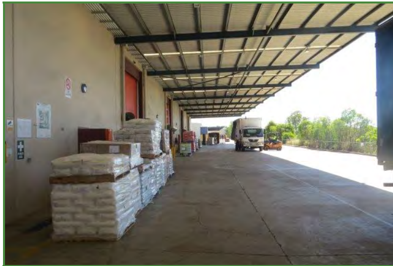
Photograph 1.6: This is a view across the front of the C warehouse and is typical of all the warehouses.
