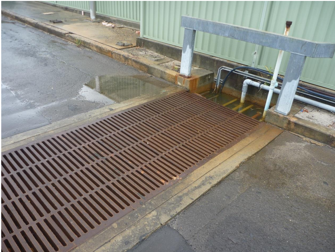
Photo 11 – Looking south, from road in Block A. Pit to be removed.
