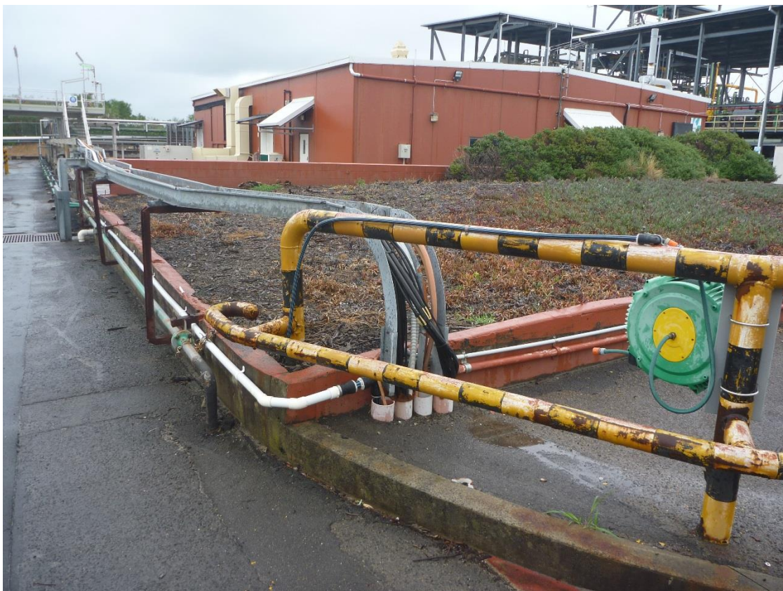
Photo 10 – Looking west, from road in Block A. Safety barrier, kerb and concrete dwarf wall to be removed by civil contractor. Pipe rack and conduits to be relocated and reinstated by civil contractor after shed is installed.
