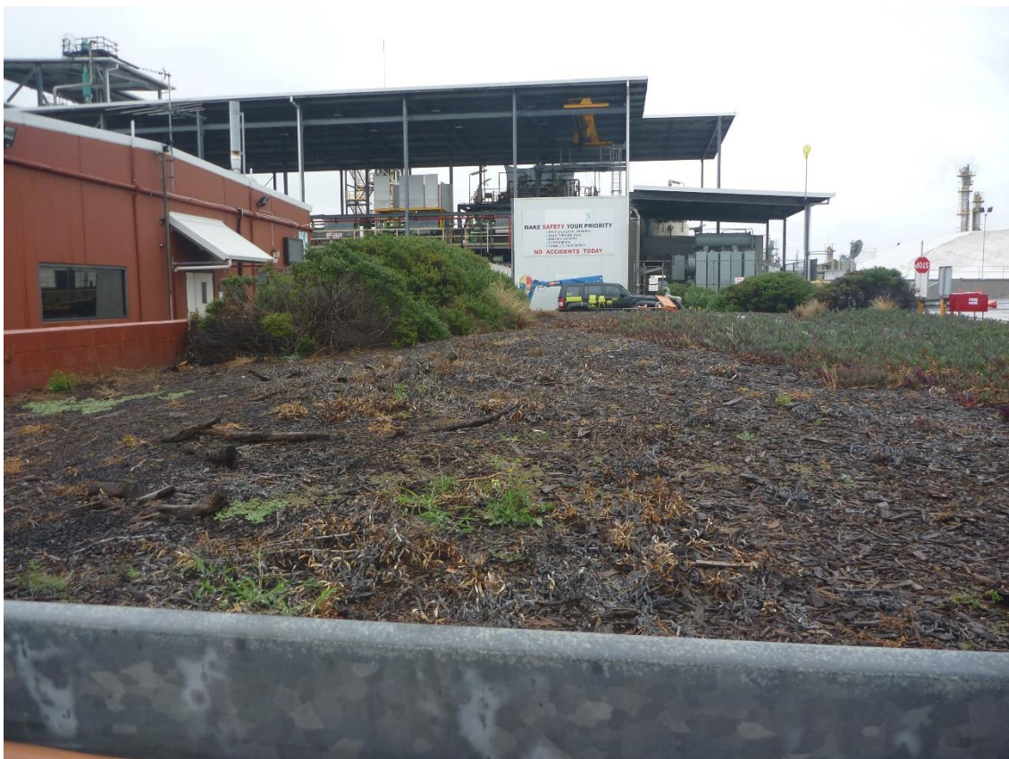
Photo 8 - Looking north-west, from road in Block A. Garden bed, soil, kerb, dwarf wall to be removed by civil contractor.
