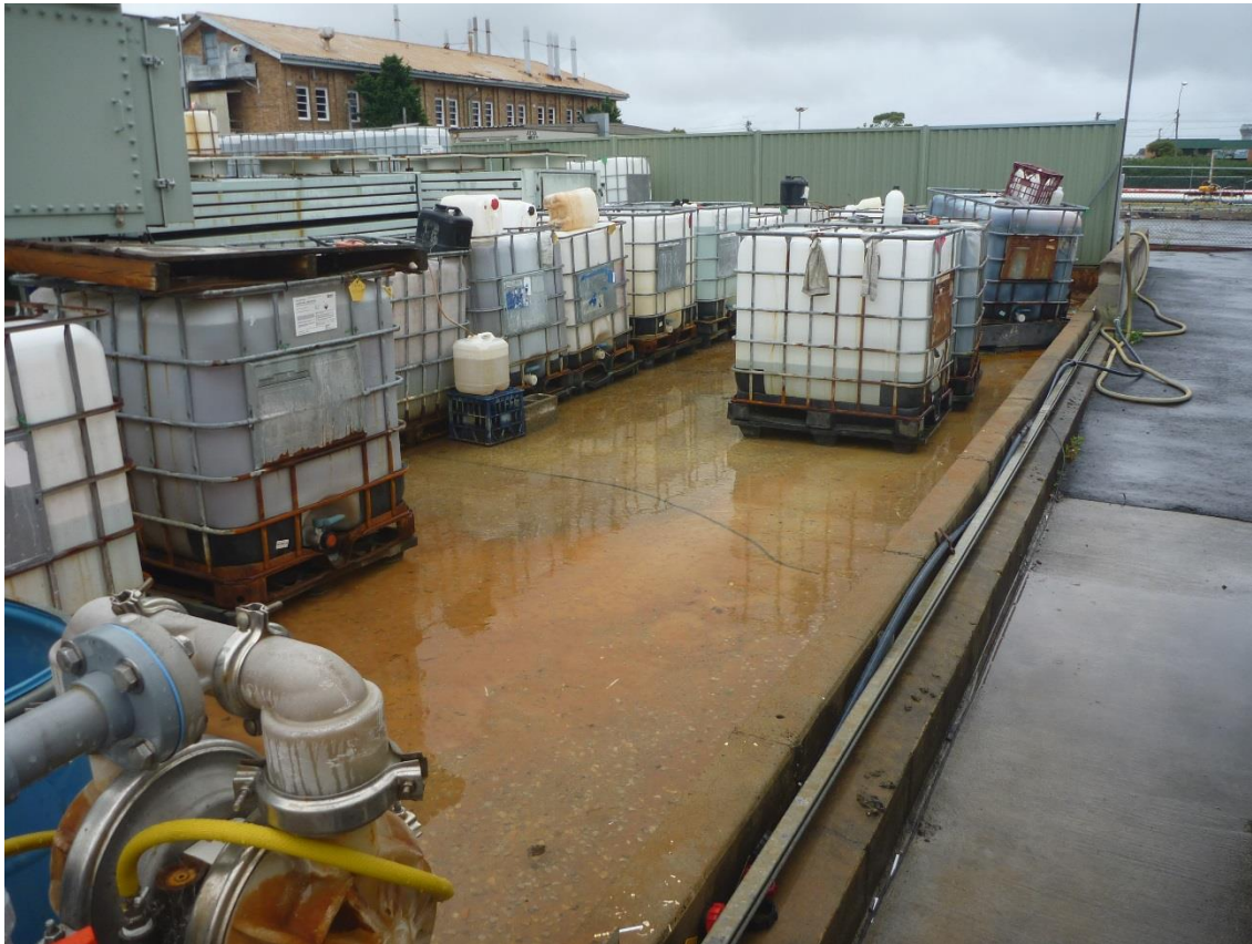
Photo 17 – Looking south-east into Memtec IBC storage area.
