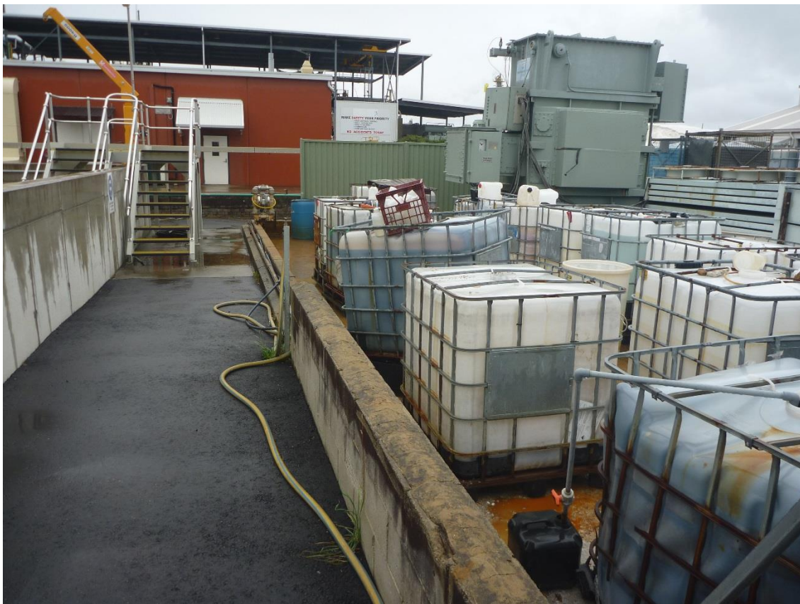
Photo 16 – Looking north-west, from west boundary of proposed Repack site. IBCs in Memtec storage area to be removed by others prior to commencement of civil works. 11kVA transformer to be relocated onto an existing plinth located elsewhere at BIP by others, prior to commencement of works. All other equipment in area to be removed by civil contractor. Bund wall to be removed by civil contractor. Green fencing to be removed by civil contractor and placed in BIP storage ( TBC ).
