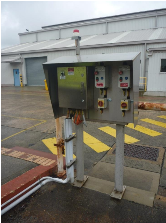
Photo 7 – Looking north-east, from Block A east boundary. Pump panel and conduits to be relocated by civil contractor.
