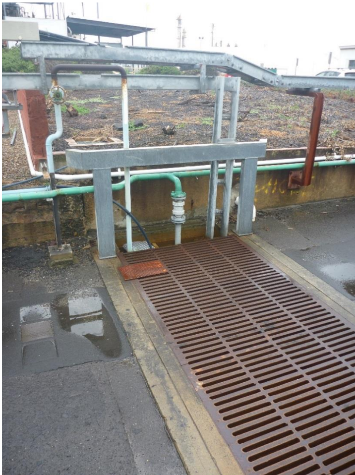
Photo 12 – Looking north, from road in Block A. Pit to be removed by civil contractor. Pipe rack and conduits to be relocated by civil contractor.
