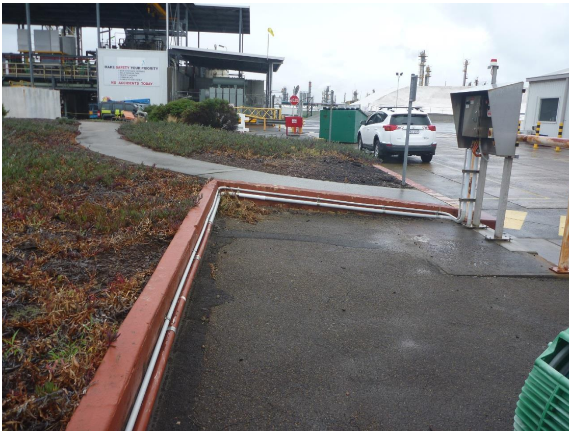
Photo 6 – Looking north-west up Block A. Pump panel & conduits to be relocated by civil contractor.
