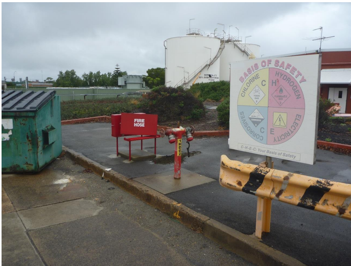
Photo 2 – Looking south from the north corner of Block A.
