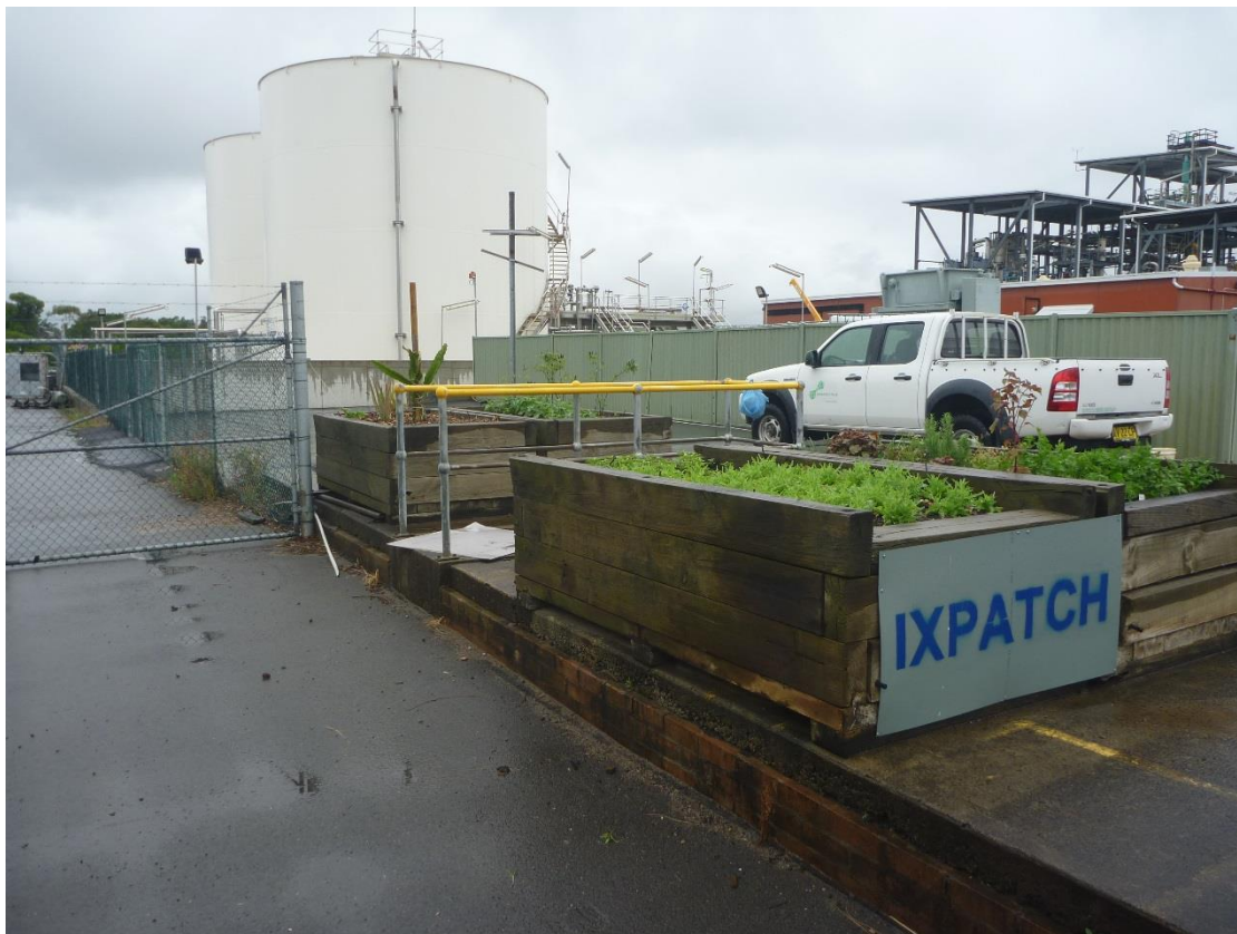
Photo 14 – Looking south-west, from southeast corner of Repack site.
