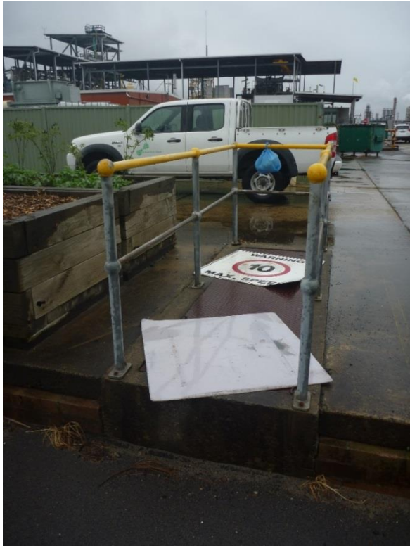
Photo 15 – Looking north, from south boundary of proposed Repack site. Underground air ventilation duct to be built up to new finished floor level ( or removed ) by civil contractor, TBC.
