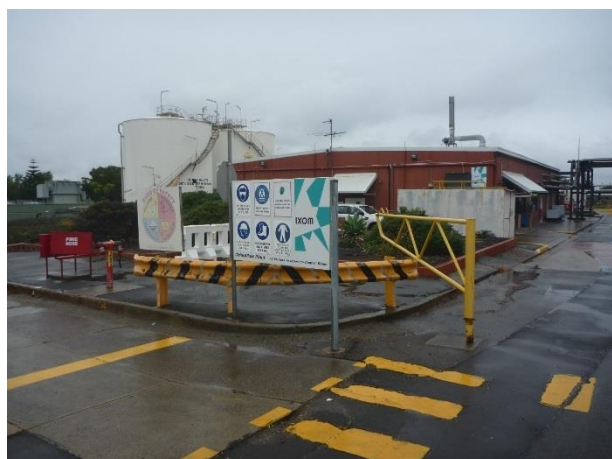
Figure 2.1 Site Context – Site Photo from North
