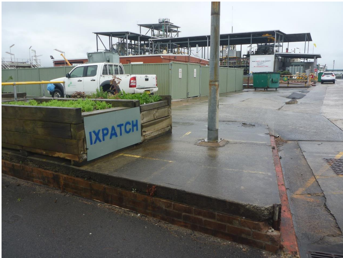
Photo 13 – Looking north-west, from south-east Corner of Repack site. ‘Ixpath’ garden to be removed by civil contractor. Light pole is outside Block A boundary and is to remain in place.
