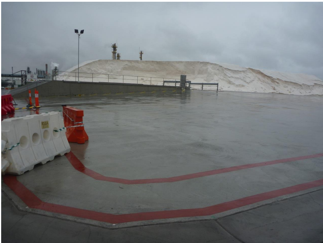
Photo 4 – Looking north-east towards new Salt Pad, from north corner of Block A. This area to be used for empty IBC storage. No modifications required to this area. Possible temporary laydown area for civil contractor.
