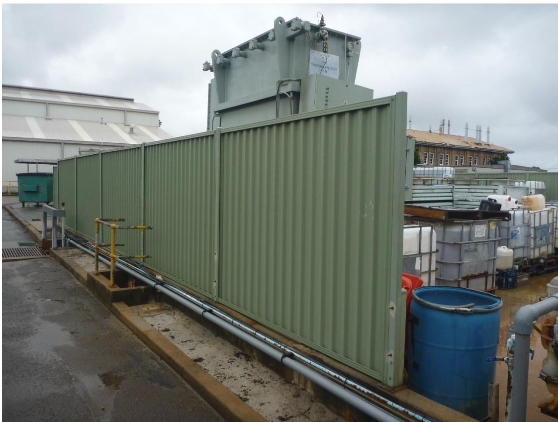
Photo 18 – Looking east into Memtec IBC storage area. Conduits to be removed by civil contractor.
