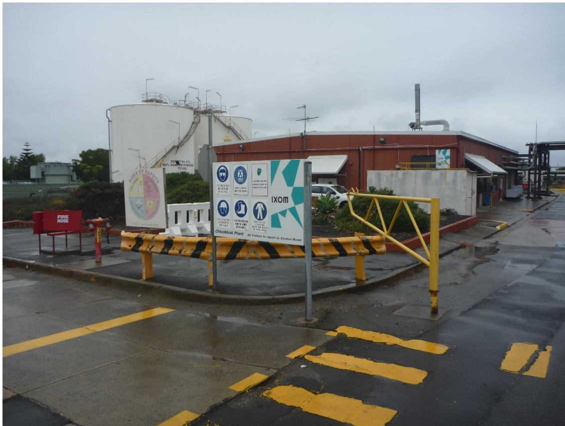
Photo 1 – Looking south-west towards existing Control Room, from north corner of Block A. Fire equipment and Ixom signage to be reinstated by civil contractor. Armco and pivoting gate to be removed by civil contractor.
