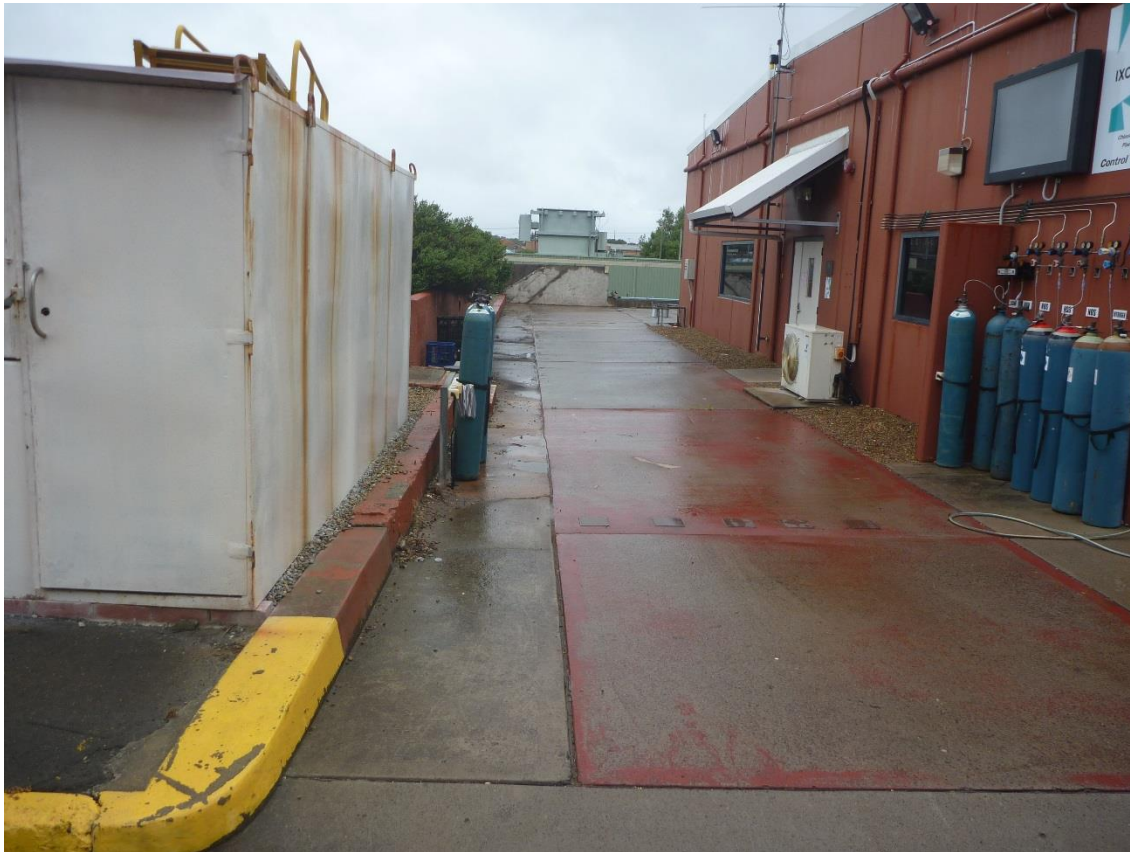
Photo 19 – Looking south-east, from north-west corner of Block A. Existing control room at right. Storage container on left to be relocated by others prior to commencement of works.
