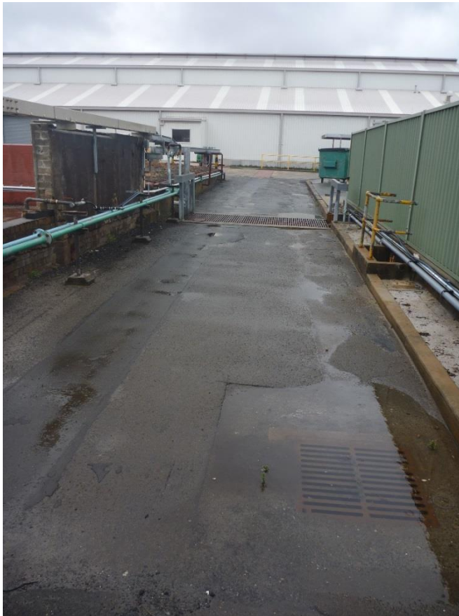
Photo 9 – Looking north-east, from west boundary of Repack site. Both pits to be removed by civil contractor.
