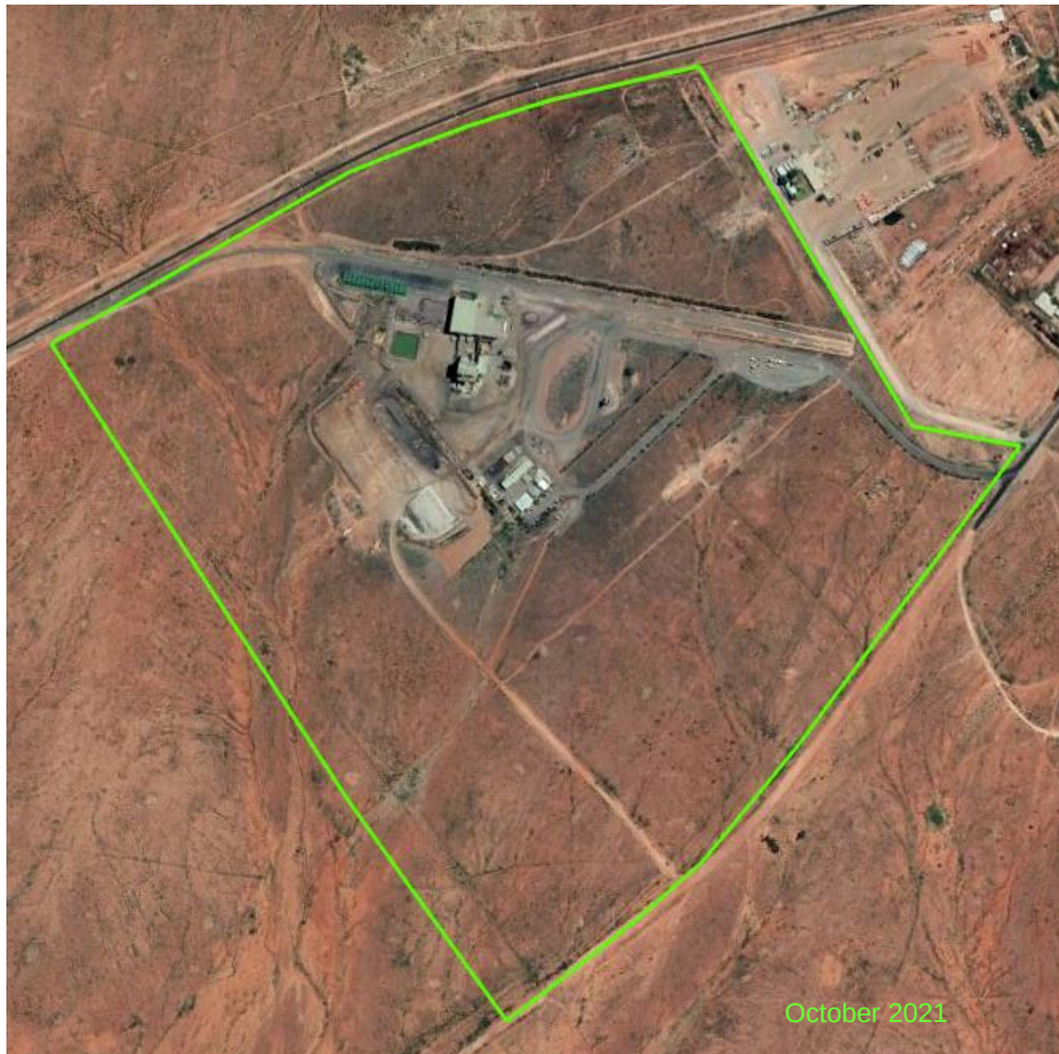
Figure 2 - Aerial Image of the MSP Plant and the Development Consent Boundary
