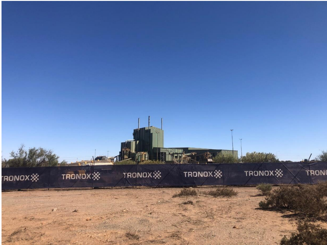
Fabric wind break installed around the site boundary
