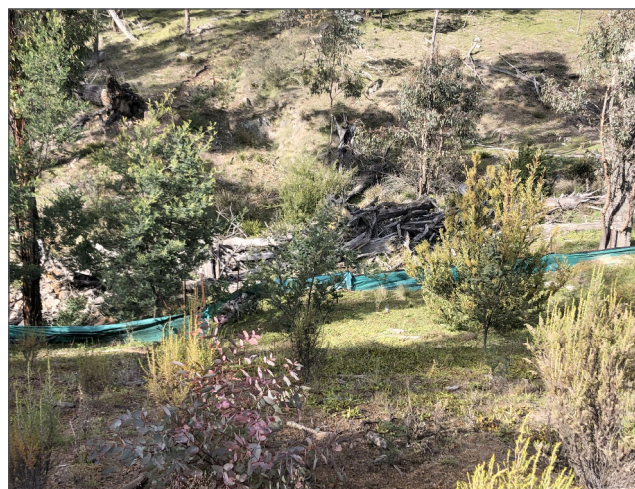
PLATE 20 Sediment Fencing (for removal)
