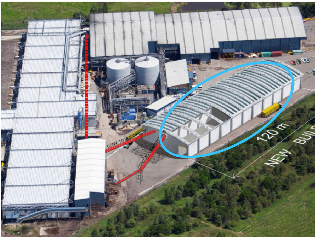
After Modification – artist's illustration showing the new OGM maturation building which also houses the PEF processing equipment
